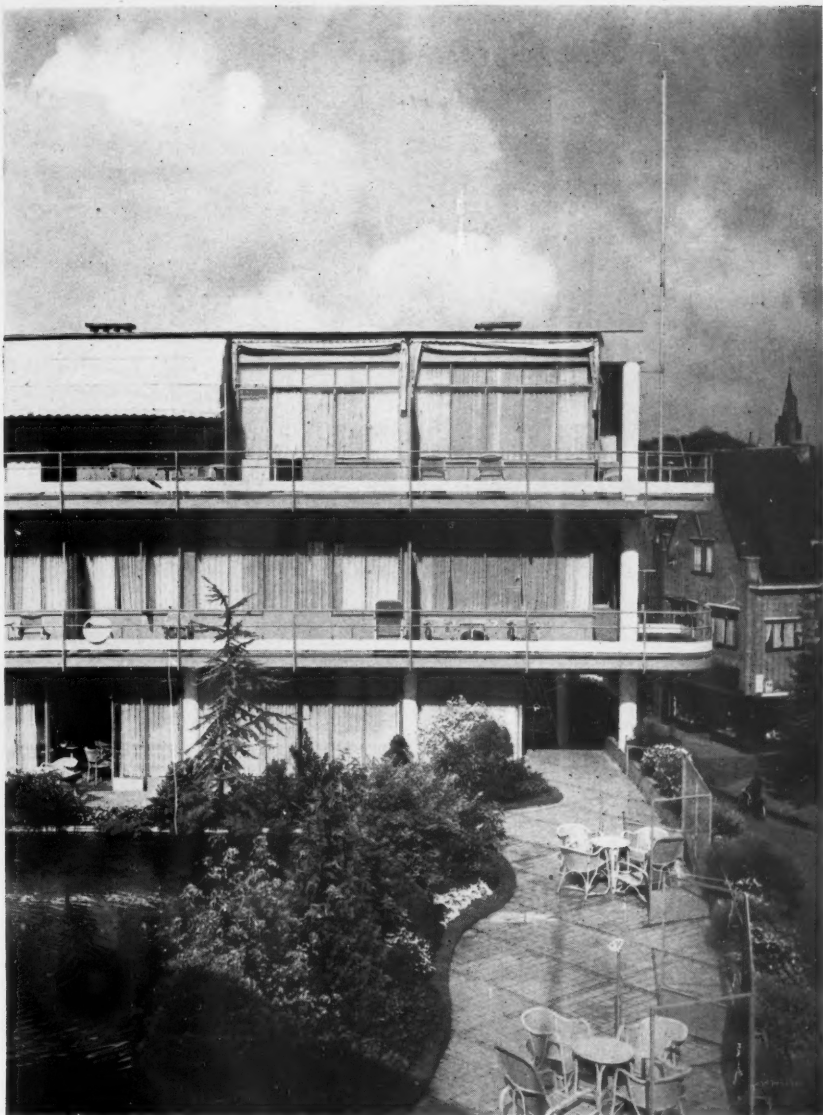
2. on opposite page, the hotel from the tree-bordered Groest; the building is faced with dull-glazed Czechoslovakian tiles. 3, the roof garden over the café and entrance hall, from one of the upper floor balconies. 4, the roof garden, from the same view point as 3, looking inwards. 5, the roof garden pool from eye level.
