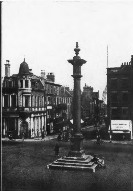
The same view in 1944. The character of the early view is retained, despite the addition of the bank on the corner.
