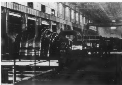
1, general view of Stourport station A from north west. 2, general view of the generating plant.
