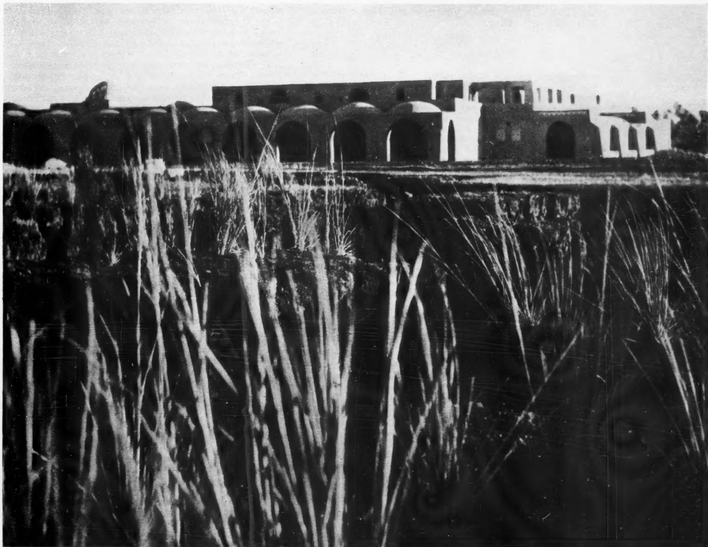
Left, simple geometrical forms produced by using mud brick in traditional Egyptian style. Below, the first section of the village to be almost completed, seen across the rough ground on which another section will shortly be built. The nearest building, with a row of small domes, is the khan or shopping centre. It is marked 2 on the general plan of the village on page 97, and shares the central village square with the mosque, the police station and the village hall.
