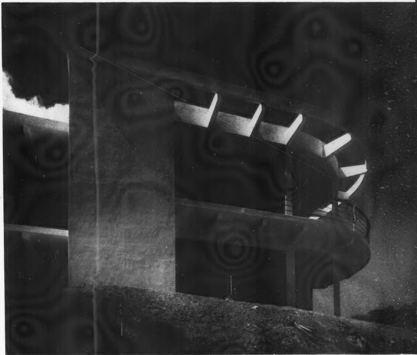
4, the living terraces from the north. Structural walls are of brick and, with stanchions and external beams, are lime-cement rendered, lime washed. 5 and 6, two views of the upper terrace.
