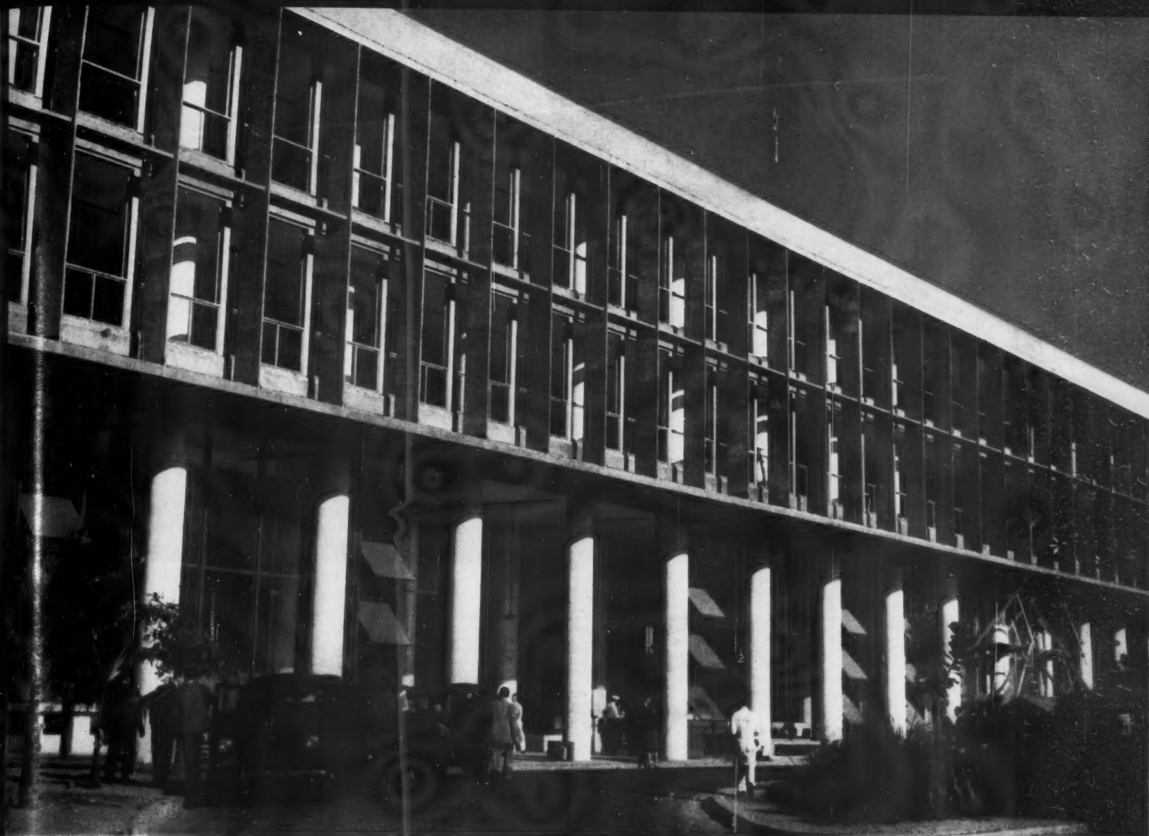
1, the entrance front which faces west. Above the ground floor this facade is protected by a brise-soleil; behind is a timber frame, still under construction, into which the sash windows and wall panels will be fitted. 2, the eastern facade onto the airfield. The control tower can be seen over the operations wing, at the near end.
