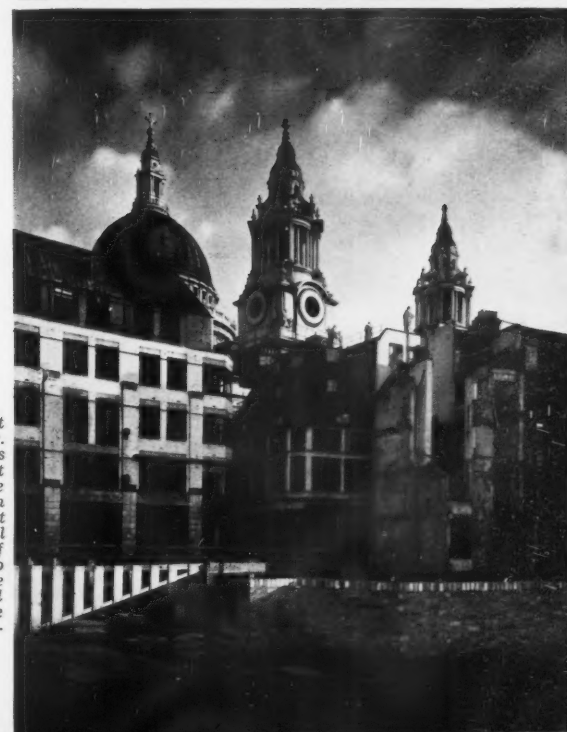
11 The dome and west towers from Amen Corner. Although the buildings screening the lower part of the cathedral have little to recommend them in themselves, their height in relation to the cathedral is just about right, and, if one closes one's eyes to details, the whole scene has the kind of visual quality which should be sought in any reconstruction of this area.
