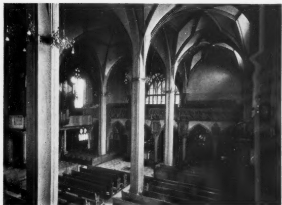
Gothic: St. Leonard's Basle, 32. Purely South German. The bays are wide, the nave and aisles of the same height, there are concave piers and net-vaults.
