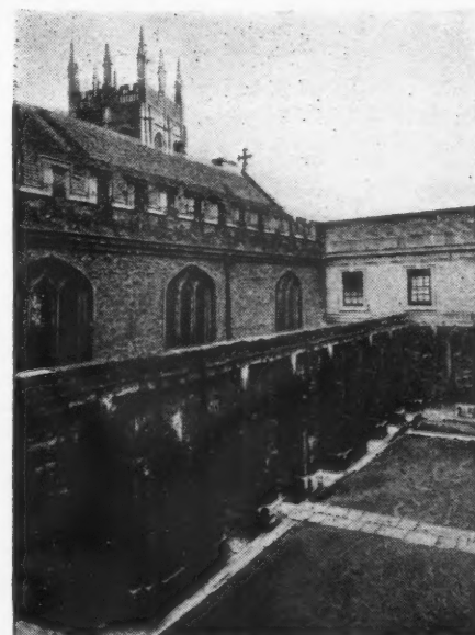
1, Corpus Christi College: cloister north of Fellows Buildings, 1712.
