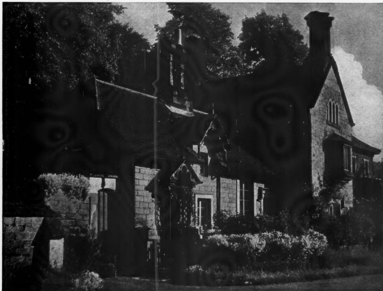
House 6—not a specially happy version of the picturesque old English cottage. The stonework of the walls is far too good, the roof is dull, the window frames are of a hopeless solidity, the trellis of the porch is miserably starved, and the barge-boarding does not get a chance to frolic as it should in a proper cottage orné.
