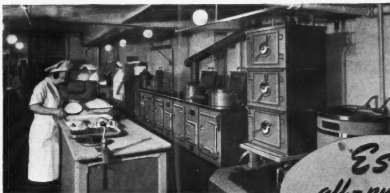
The kitchen of Messrs. Sainsbury Ltd., London, showing a line assembly of ESSE Major Cookers used in conjunction with ESSE Steam Heated Equipment
