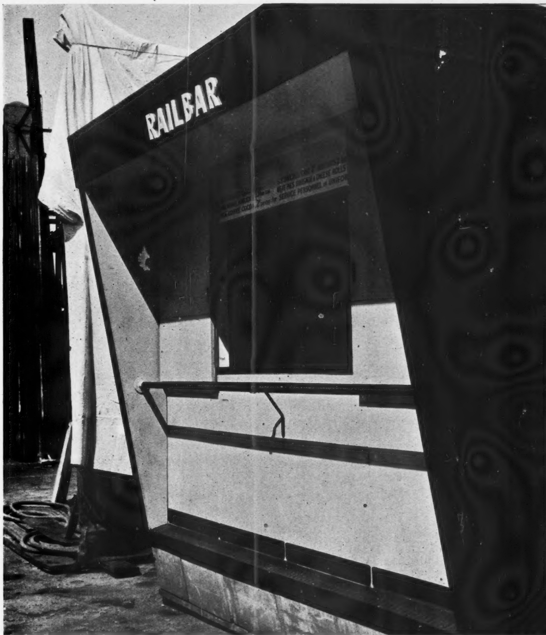
base units fixed, back unit fixed, end unit being placed in position
