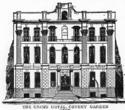
Russell House, No. 43, King Street, Covent Garden, designed c. 1705 for Admiral Russell, the victor of La Hogue. The coarse Corinthian pilasters on the high plinths and the attic surging up in the middle are typical Archer features. The building became later Evans Grand Hotel, the Cave of Harmony of Thackeray's The Newcomes . It housed the Institute of British Architects, 1835-1837.
