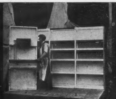
base units fixed, back unit fixed, end unit being placed in position
