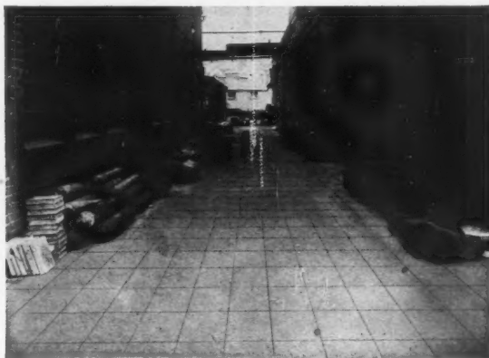
Ferrogran Flag Flooring in a passage way at a Stampings Works
