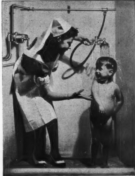
Leonard-Thermostatic Hot and Cold Water Mixing Valve serving a shower at a Day Nursery
