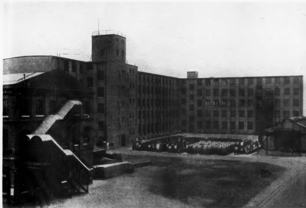
1912 Building with skeletons of steel or reinforced concrete when it was first introduced into this country, had no æsthetic appeal to architects. It was either used in a straightforward, convincing way by engineers for factory buildings such as the Siemens's rubber workshops at Woolwich of 1912, 7, or hidden behind heavy masonry and sumptuous decoration, as in the Morning Post by Mewès and Davis of 1908, 8. To-day the greater honesty of the concrete factory makes us overlook the fact that its appearance was probably to a much lesser degree the work of conscious proportioning and balancing than we expect.
