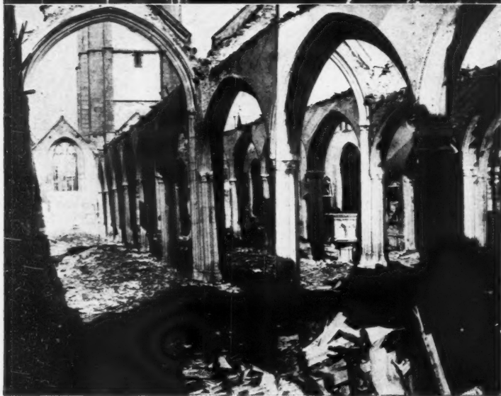
ST. ANDREW'S CHURCH stands in the centre of Plymouth, its roof and furnishings burnt and its monuments badly damaged. It is a grand early 15th century building, with aisles running the whole length and short additional aisles on north and south giving a transeptal effect on plan. The dominating west tower was built at the expense of a Plymouth merchant in 1440-60. Granite has been much used, particularly in the beautiful arcade capitals and the dressed masonry of the tower. The fine effect of the arcades and continuous barrel roof is well seen in the engraving, taken shortly after Foulston's remodelling of 1826. The church was taken in hand by Sir Gilbert Scott in 1874-5 and Foulston's work, with other Georgian features, removed. The monuments in St. Andrew's are of great interest and range from elaborate 16th and 17th century mural monuments to the bust (slightly damaged) of Dr. Zachariah Mudge, executed by Chantrey from a painting by Reynolds. Adjoining the church is the medieval Prysten House which has been badly damaged though not burnt.
