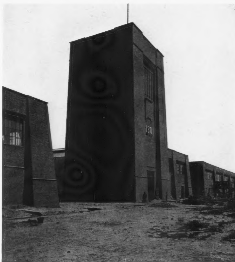
1901 H. Bulkeley Creswell's Queensferry Factory, 1, the most advanced British building of its date. Why is it not just as famous as Peter Behrens's turbine factory of 1909?
