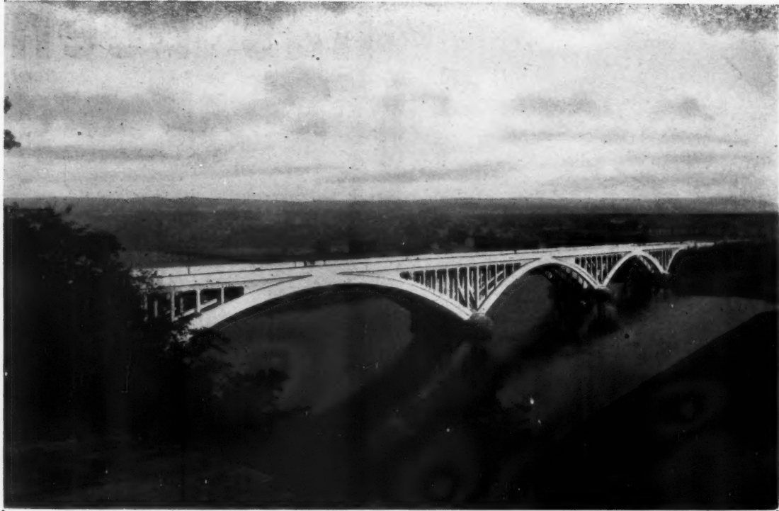
The Royal Tweed Bridge, Berwick, completed in 1928, has a total length of 1,398 feet.
