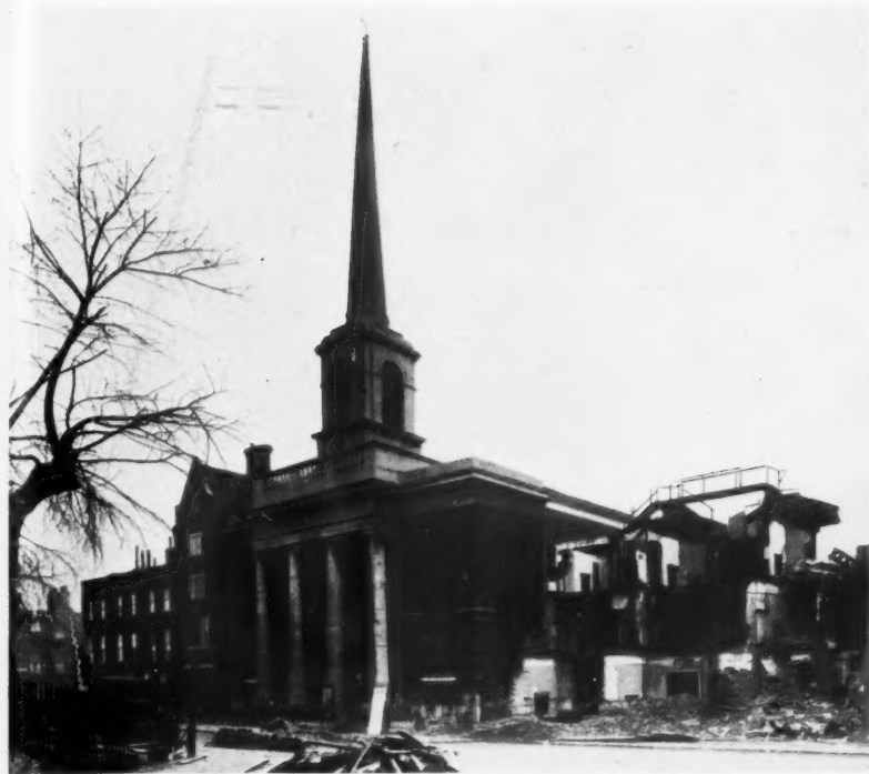
ST. BARNABAS, KING SQUARE, FINSBURY , was designed by Thomas Hardwick, the surveyor to the St. Bartholomew's Hospital estate on which King Square stands. It was one of the churches built under the Church-building Act of 1818 and was begun in 1822. This was the same year as All Souls, Langham Place, so it is impossible to guess whether Hardwick or Nash was first with the idea of a short, needle-pointed spire raised over an Ionic portico. Hardwick had already built several London churches, including St. John's Wood and St. Marylebone. He was an old man in 1822 and, as a pupil of Chambers, had always held conservative views; so the character of the King Square church may well be due to his son Philip, of Euston Arch fame. The badly wrecked interior of the church was of the plainest possible type. The excellent but inappropriate gabled vicarage on the left is by James Brooks.
