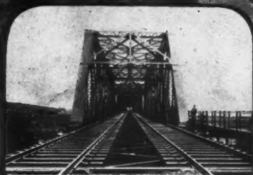
Teak sleepers on the Nerbudda Bridge, India, exposed to vibration, sun and rain.
