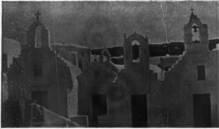
5. A row of independently built chapels on the island of Mykonos, set up as ex voto offerings by sailors delivered from shipwreck. These chapels, of which there are many on the island, are all barrel-vaulted in contrast to the flat roofs of the dwelling houses. Excavated churches and houses are not seen on Mykonos, and are indeed quite special to the Isle of Santorin (or Thera), whose volcanic rock lends itself to such treatment; nor are barrel-vaulted houses seen on any other island but Santorin.
