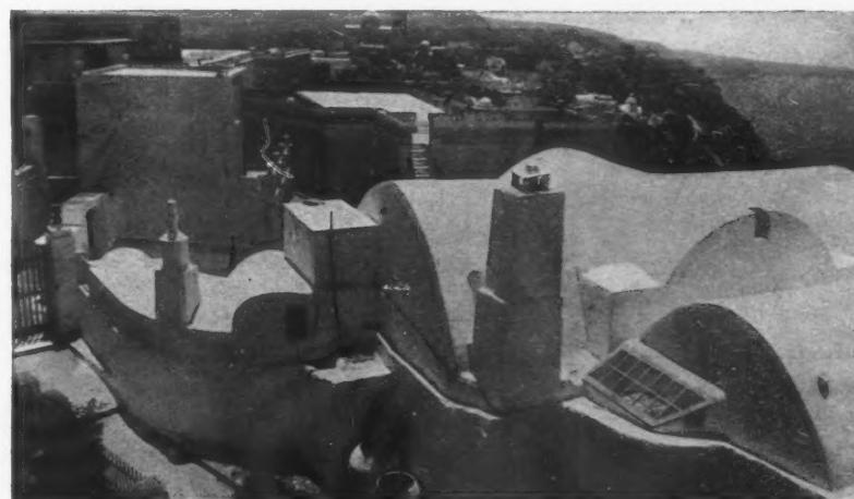
4. In the foreground is the roof of the hotel at Thera, an excellent modern example of the traditional method of roofing employed on Santorin. Volcanic pozzolano is used and sets so fast that in an hour or so the roof can be walked on. Barrel vaulting stands up against earthquake shock far better than flat roofs, also seen on this island.
