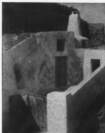
2, a peasant's house at Santorin, hollowed out in volcanic rock: porches and walls have been added. The householder hardly ever owns the land over his own roof, but he has the right to veto certain uses to which it may be put. 3, the harbour at Santorin and rock-hewn houses and churches with façades built on. Some troglite churches and houses, carved out of the friable volcanic cliffs, can also be seen.
