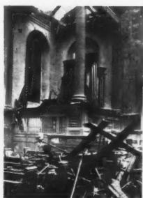
ST. ANNE AND ST. AGNES, GRESHAM STREET , has been severely damaged, though not destroyed. Built by Wren after the Great Fire, it is one of the "greek cross" churches, and the interior, with four columns carried on very high pedestals, is especially successful. The exterior, whose red bricks have at some time been covered with stucco, is less satisfactory.
