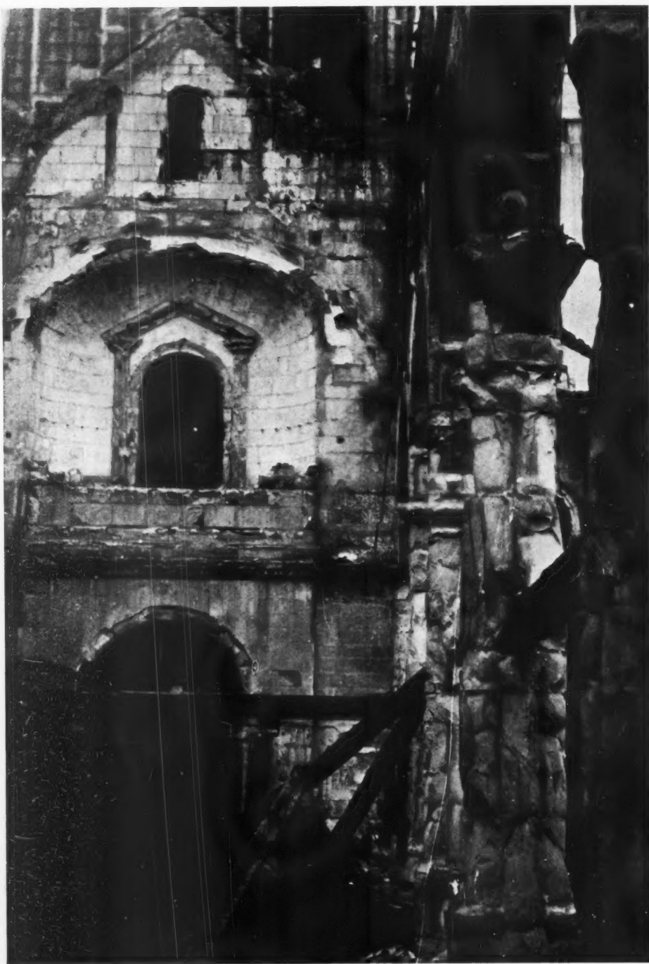
Another detail of St. Bride's, Fleet Street. The west wall of the burnt-out nave showing the characteristic texture. A night of fire has the effect of centuries of weathering.
