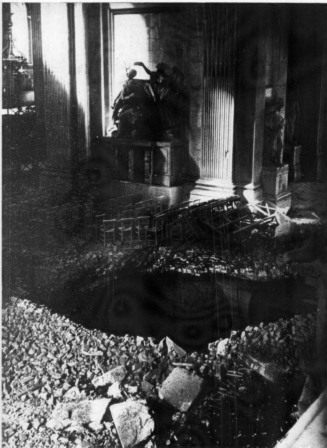
The view (left) in the north transept of ST. PAUL'S CATHEDRAL , shows where the debris brought down by a bomb caused the church floor to collapse into the crypt. The large monument against the pier, damaged by the explosion, is to Admiral Lord Rodney and is the work of Rossi. The standing figure against the end of the pier is Earl St. Vincent, by Baily. Among the debris can be seen remains of the portico to the north door. It is fortunate that neither of the direct hits which the cathedral has received have interfered with the stability of the structure as a whole, having merely pierced the light coverings between main points of support.
