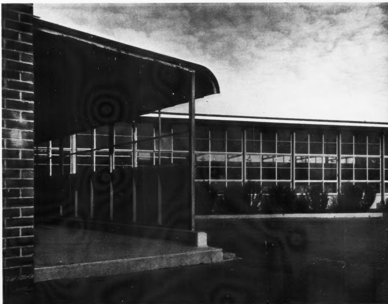
5, the rear classroom wing, containing the handicraft and science room with, in the foreground, the open end of the main classroom corridor. This photograph well illustrates the nature of the classroom construction which is of light steel sections designed to be semi-permanent only, with a view to future alteration to suit changing needs. The corridor is of similar construction with permanent ventilation contrived beneath the overhang of the roof.
