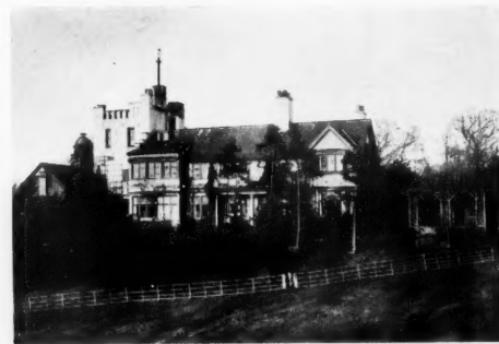
Watt's first building enterprise, his own house designed for him by Henry Brooks in conventional Cheshire Style. The tower was added by Watts himself when he built his other houses after working out his own original style.
