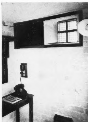
WARDENS' POST—Here four P.B.3 Glass Bricks have been built into the wall to give natural lighting. A shutter slides across at night.
