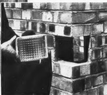
TRAFFIC WARNING LIGHTS can be provided at the corners of shelters which jut into the roadway, by the insertion of glass bricks. The smaller photograph shows how the brick is fixed in. Illumination comes from within the shelter.
