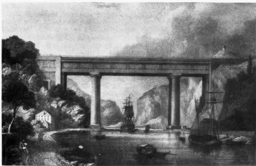
PROPOSED PLAN OF A BRIDGE ACROSS THE AVON FROM ST VINCENT ROCK TO LEIGH WOODS. The bridge is to be of stone, and is to be of the following dimensions: Length of bridge 1,000 feet Width of bridge 40 feet Height of bridge 20 feet The bridge is to be of the following dimensions: Length of bridge 1,000 feet Width of bridge 40 feet Height of bridge 20 feet
