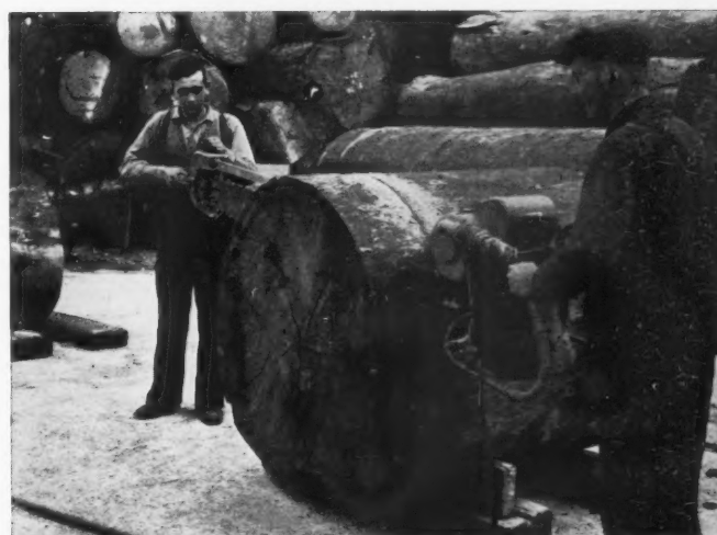
Gaboon logs being cut to length with portable electric chain saws ready for passing to the rotary cutter or "peeling machine."
