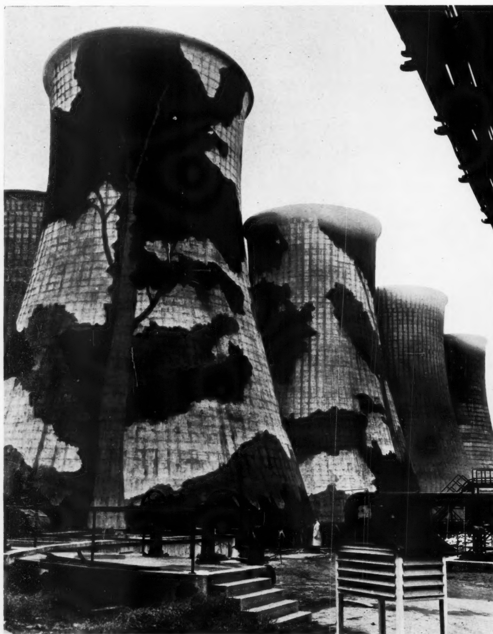
The cooling towers of the central generating station of the Leicester City Electricity Service which have recently been camouflaged. The tone and colour values of the design match the trees and fields which surround the station. The towers are 120 ft. high and over two tons of special oil bound water paint was used on each. The scheme was prepared by Mr. Ernest Townsend of Derby.
