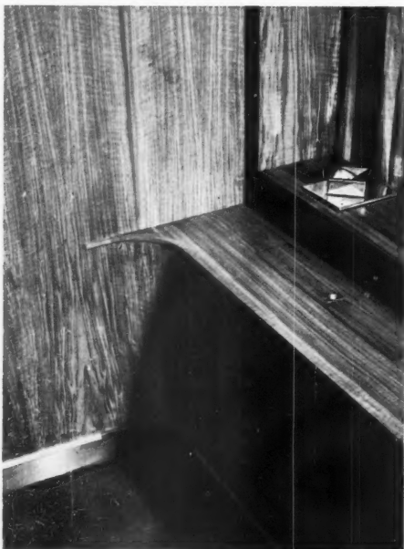
Plywood as a backing for veneers
