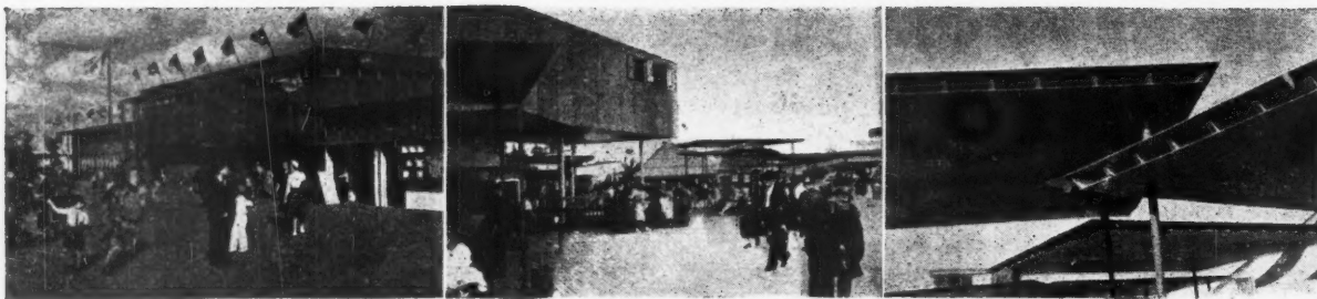
Three typical views in the Children's World, showing the appropriate simplicity and spaciousness of the buildings and layout. George Howe, architect.
