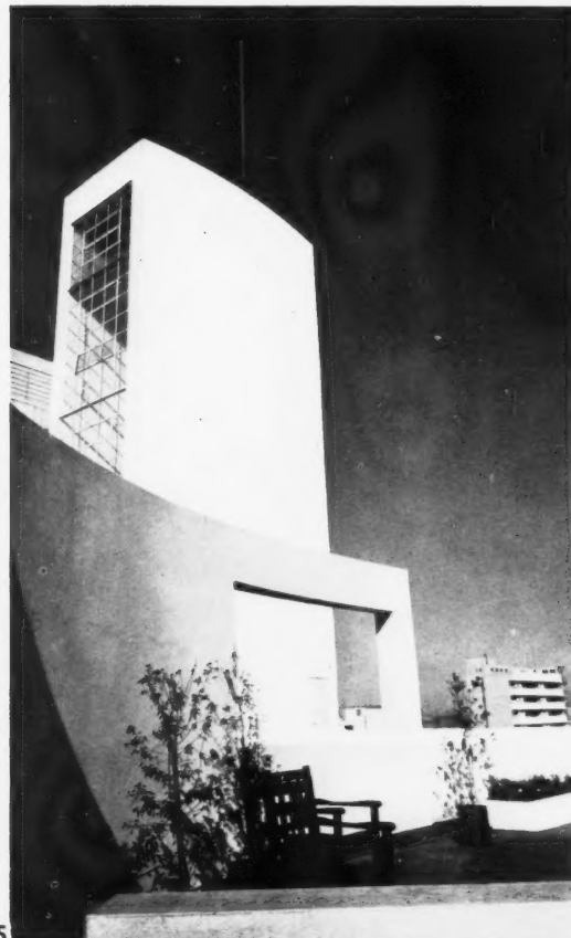
4, detail of the stair tower with the lift well to the left. The open, horizontal-railed balconies on the right serve the flats. The balcony rails are painted a chocolate colour, with the flat doors in cerulean blue. 5, view from the roof terrace. The curved screen wall, in the left foreground, is colour washed a pale green with the staircase tower beyond in cream-white.
