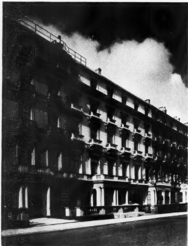
Part of Leinster Gardens, Bayswater. In the middle of the picture are the two houses, numbers 23 and 24, which are only dummy façades. See the note on this page.
