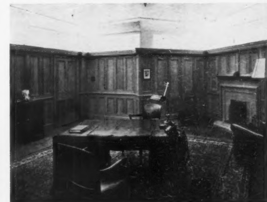
CORNICE LIGHTING IN A PRIVATE OFFICE. Lamps spaced at 3 ft. intervals.
