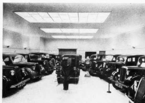
LAYLIGHTS IN A MOTOR SHOWROOM. Architects : Allcock & Grieves, F.L.R.I.B.A.
