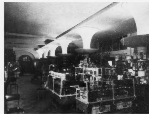
INDIRECT PILLAR LIGHTING IN A STORE. Architects : Stonebridge & Harris, F/L.R.I.B.A.
