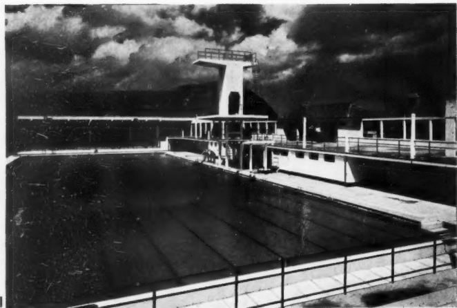
1 and 2, the Minehead Swimming Pool; Edwin Gunn, architect. Separate space for about 600 spectators is provided on tiers and terraces with possible supplementary space for gala occasions.
