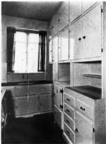
Kitchenette at Barrie House, Lancaster Gate. The built-in cupboards and dresser are of plywood construction cellulosed a cream-white. The refrigerator is incorporated in the cabinet fixture. Architects—Howard Leicester & Partners. Contractors—Rota Products Ltd.
