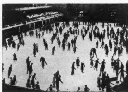
A first step in the direction of the comprehensive recreation centre is found in the subsidiary attractions provided in the pub. A second is the provision of multi-purpose buildings such as the Wembley swimming pool. The illustrations on the left show the building converted to serve three distinct functions: swimming, tennis and skating.
