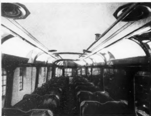
INDIRECT LIGHTING FROM UNITS ABOVE THE WINDOWS IN A TRAMCAR.
