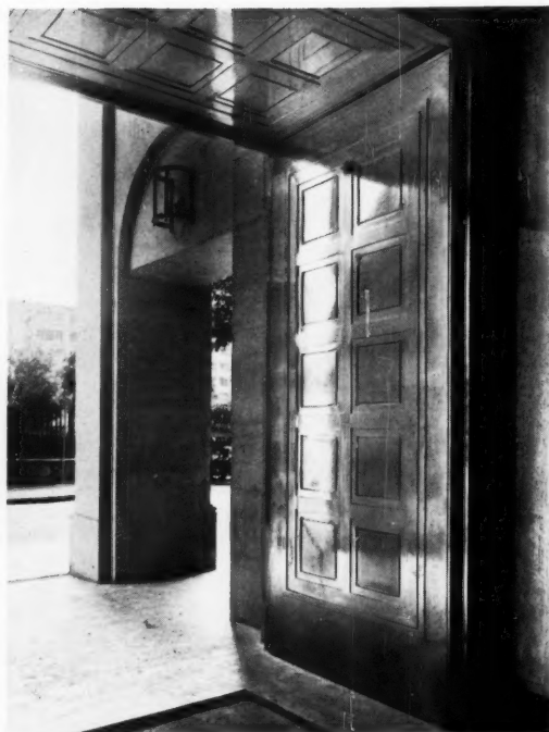
The entrance doors and soffit to Dean Bradley House have been executed in extruded nickel silver (20% nickel). Architects: Wimperis, Simpson and Guthrie. Craftsmen: J. Starkie Gardner, Ltd.
