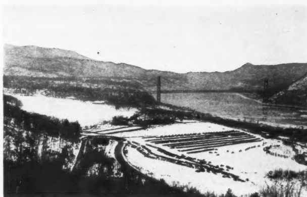
An obstacle often put forward as precluding the development of National or Regional Parks is that the areas involved will often overlap the districts controlled by a single authority. That this difficulty can be successfully overcome is shown by the case of the Palisades Interstate Park, which is administered jointly by commissioners representing the States of New York and New Jersey. Special features of the Park, which is in reality formed of a chain of parks equipped for all forms of recreation, are the indoor and outdoor museums maintained by the Park in co-operation with the American Museum of Natural History. On the left are winter and summer views of one of the Parks, the 1,000 acre Bear Mountain Park, which is specially equipped as a winter sports centre.
