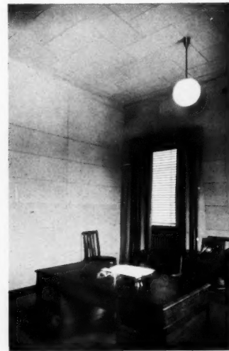
The new Celotex Offices: architect, Septimus Warwick. Left, the staircase-hall. Ceiling, walls, dado and carved relief panels are in "Celotex" insulating board and "Texbord." In the executive office, right, "Celotex" tile-board provides the ceiling finish, and insulating board with a natural sanded finish, in the form of bull-nosed units, is used for lining the walls.
