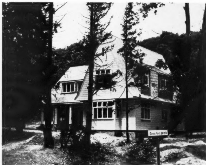
A timber house at Caterham, Surrey, designed by R. V. Boughton and constructed under the supervision of the Timber Development Association.
