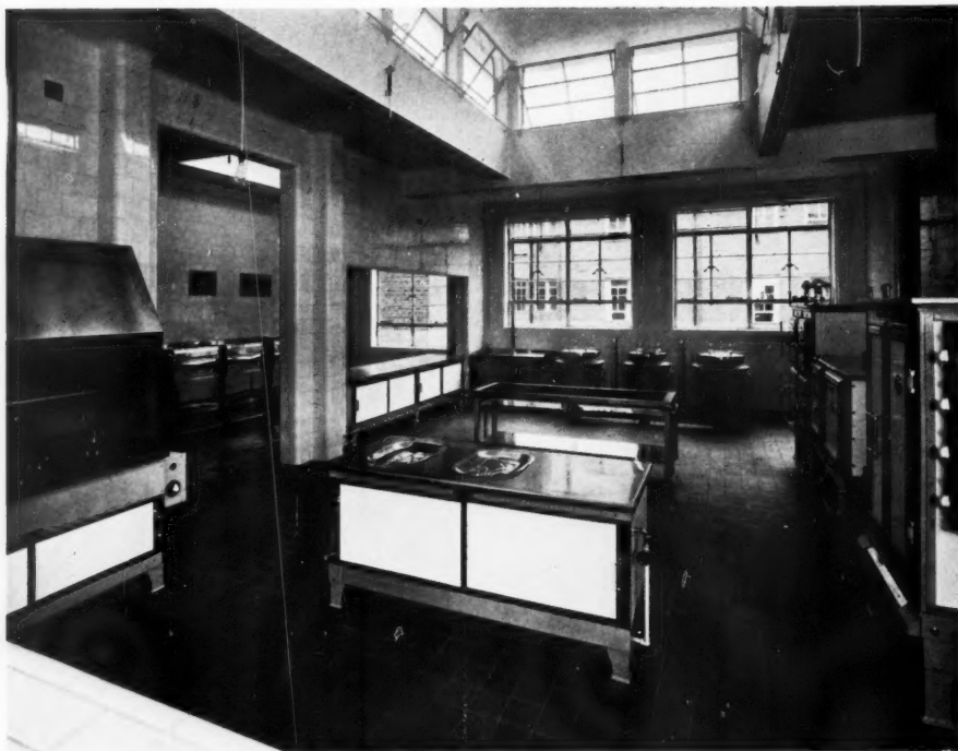
Kitchen at the Redhill County Hospital, Edgware. The walls and floor are tiled; the equipment is of special finish which comprises an extensive use of stainless steel, chromium plating and vitreous enamel. Surfaces that are easily kept clean are an essential in the modern kitchen. Architect—W. T. Curtis. Contractors—Benham & Sons Ltd.
