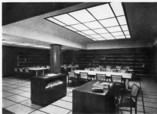
LAYLIGHTS IN A UNIVERSITY LIBRARY. Architect : Harold A. Dod, M.A., F.R.I.B.A. (Willink & Dod).
