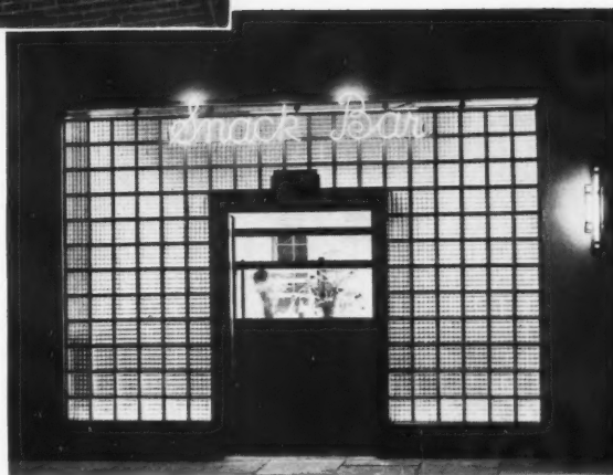
Left: Snack Bar Entrance. Designed by Eric Thompson. Builder: A. G. Scott, Ltd., E.C.4.
