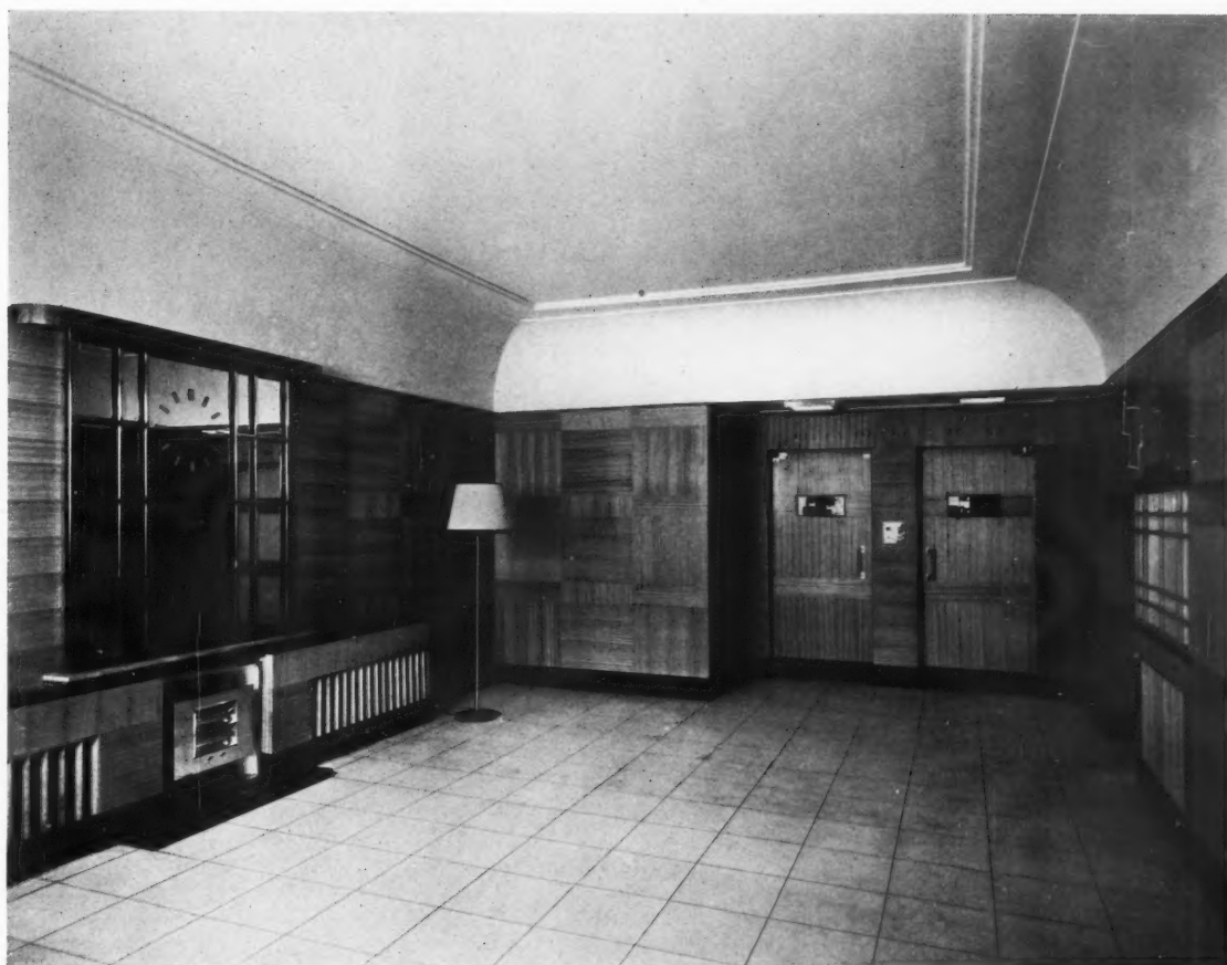
St. John's Court, Finchley Road, N.W.3.
