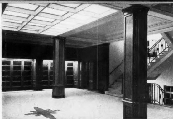
LAYLIGHTS IN AN ENTRANCE HALL. Architects : Howard & Souston, F.R.I.B.A., F.S.I.
