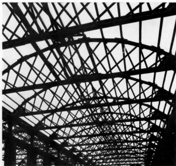
Pattern in timber. An example of all-timber roof construction.
