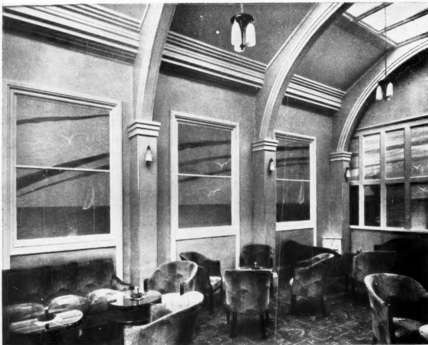
Ladies' Lounge of the Royal Hotel (LNER), Grimsby. Art "Thermolux" windows designed and installed by James Clark & Son, Ltd.
