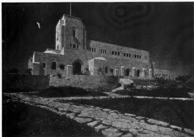
Quite distinct from the modern, often experimental, character of the majority of buildings reviewed here, is the more official style generally adopted for government architecture. Above, the Palestine Archeological Museum at Jerusalem, built on a site at the extreme eastern end of the north wall of the old city. The view is taken looking across the museum towards the Mount of Olives. The building was designed by the former government architect, Austen St. B. Harrison with Paul Manger and William Price of the Palestine Public Works Department as assistants. Below, Government House, Jerusalem: the north-east front. Austen St. B. Harrison, architect.
