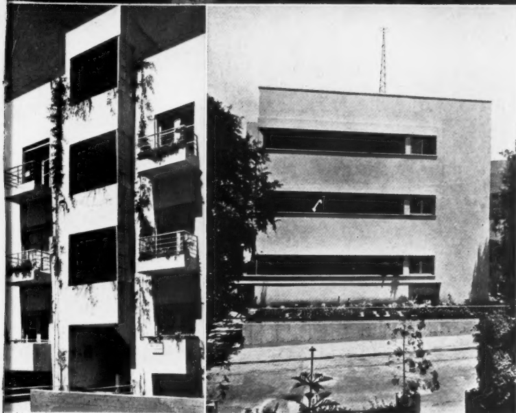
Left, workers' co-operative flats in Tel-Aviv, A. Sharon, architect, embodying the principles of east-west cross ventilation and terrace balconies which are applied throughout the design of these buildings. Right, a block of flats on an irregularly shaped site in Tel-Aviv. D. Karmi and Z. Barak, architects. There are two flats on each floor: each with living-room, dining-room and two bedrooms.
