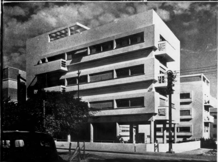
An apartment house in Tel-Aviv containing 15 flats: Z. Rechter, architect. The greater part of the ground floor is open, and planted as a garden. The illustration shows the main elevation of the building.
