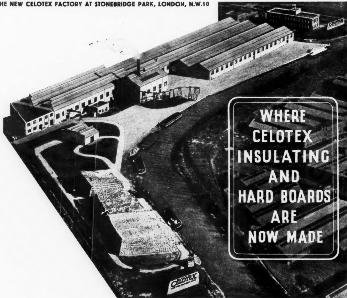
THE NEW CELOTEX FACTORY AT STONEBRIDGE PARK, LONDON, N.W.10
