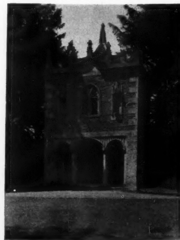
A pavilion by "Capability" Brown at Corsham Court. The pinnacles and stained-glass windows are said to have been added by Nash.
