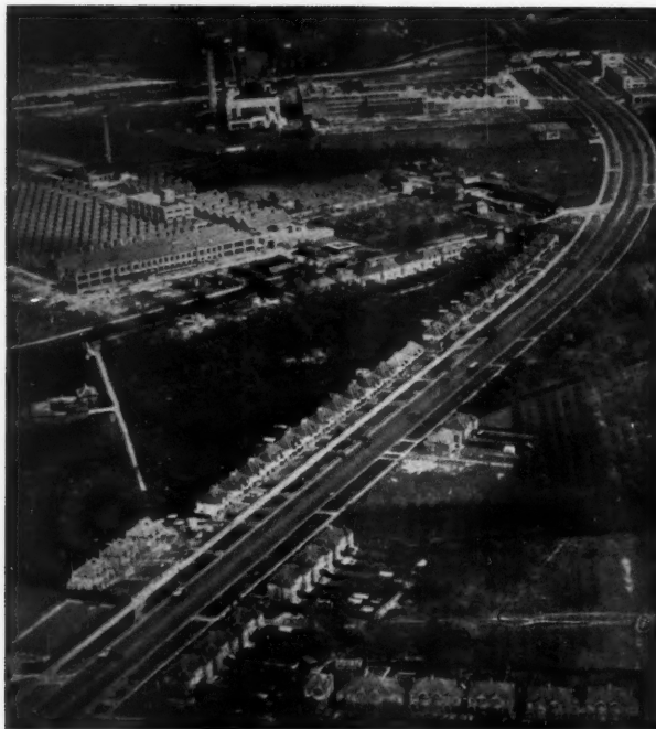
The Great West Road, a bad example of ribbon development and of indiscriminate mixing of domestic and industrial building.
