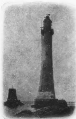
The present Eddystone lighthouse, completed in 1884. It is largely modelled on Smeaton's design, which it superseded. The remains of the latter can be seen on the left, looking like its tree-stump prototype: see facing page.
