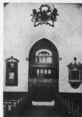
Richmond Church, Surrey, an example of "intelligent" restoration illustrated in "The Protection of our English Churches" (see note on this page). Above is the west end as it was: "Mediaeval tower arch blocked by worthless modern gallery, royal arms dismembered, monuments skied." Below, as it now is: "Tower arch exposed, royal arms repaired, monuments lowered and cleaned."
