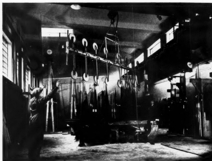
"Sucker Gear" in operation. The plate of glass being lifted weighs approximately 8 to 9 cwt.
