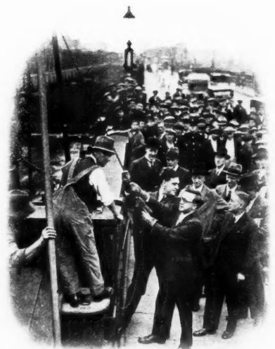
Mr. Herbert Morrison performs a ceremony: lifting the first stone to inaugurate the work of destroying Waterloo Bridge. 14
