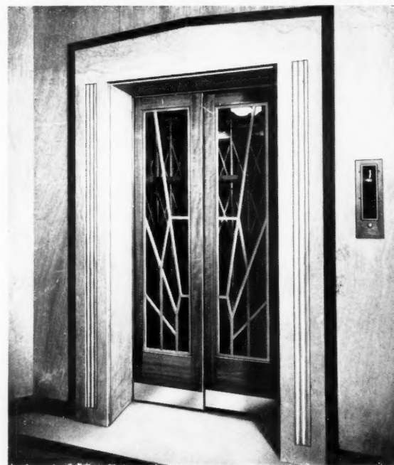
The delicate Grilles forming these lift-doors are castings in 'AERIAL ALLOY'—EACH BEING CAST IN ONE PIECE . . . BY
