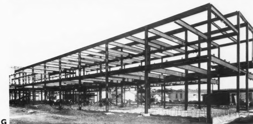
D, STEEL CRAFT HOUSE. Prefabricated bathroom, showing combined plumbing for bathroom, kitchen and porch. E, PLYWOOD MODEL HOUSE, LOS ANGELES, CALIFORNIA. Garden view. F, SUPER-PLYWOOD MODEL HOUSE, LOS ANGELES. Night view seen from patio, with collapsible glass partition opened. G, RALPH WALDO EMERSON JUNIOR HIGH SCHOOL, LOS ANGELES. One of the first earthquake-proof steel skeletons used in the Los Angeles school district. The effort to clearly establish internal stresses caused by the lateral forces of earth shocks and wind attacks favours the use of fabricated steel skeletons even for one- and two-storey school buildings in California.
