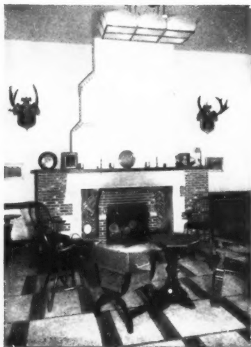
"Semi-indirect lighting fittings are employed in this Norman style apartment."
