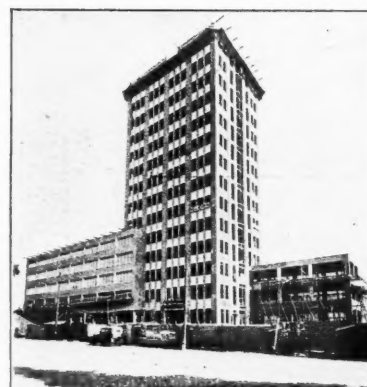
Municipal Electricity Works, Rotterdam (Holland)
