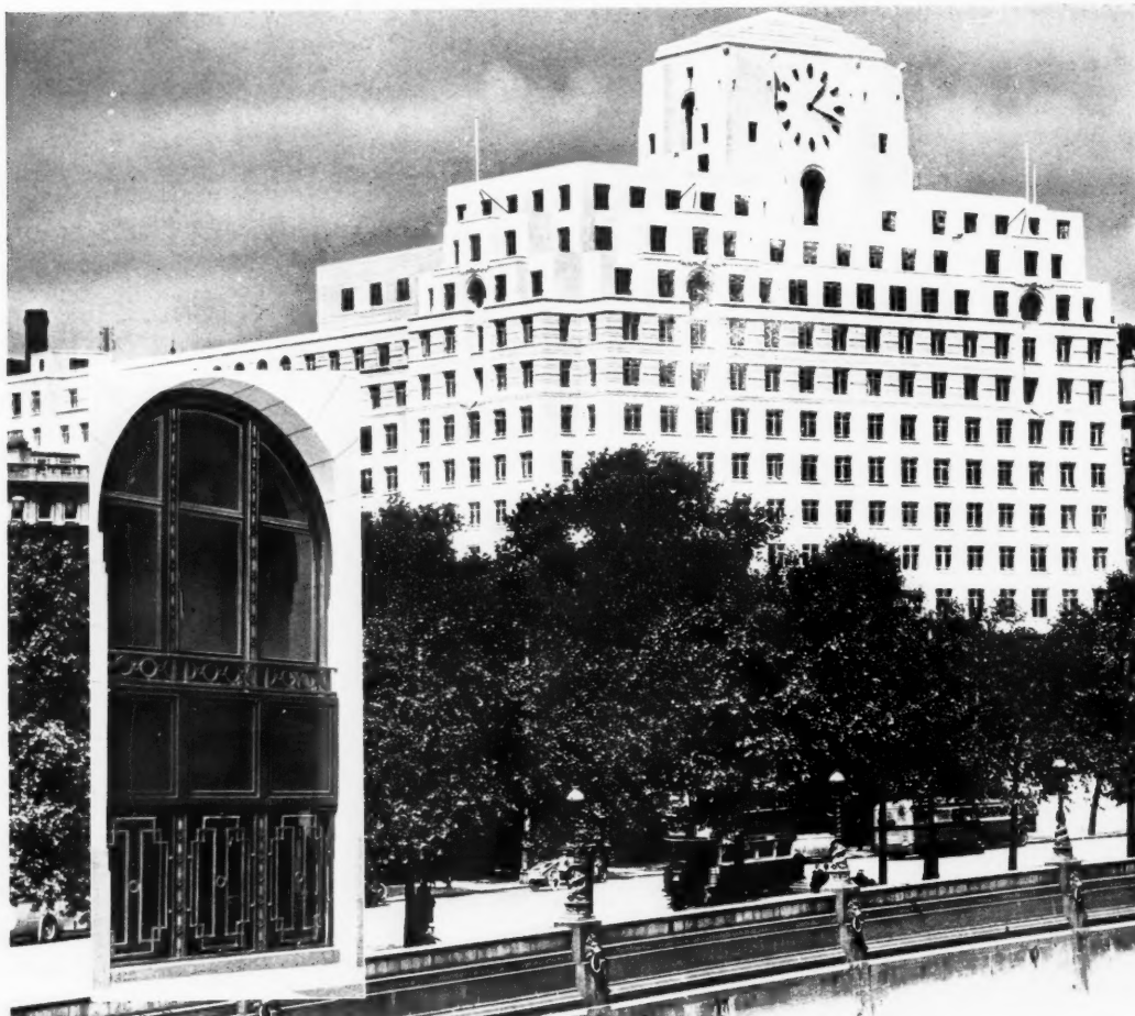
CAST IRONWORK, AS INSET ILLUSTRATION, ALSO BUILDING FRONT PANELS AND RAILINGS, SUPPLIED AND ERECTED AT SHELL-MEX HOUSE, LONDON. ARCHITECTS: MESSRS. JOSEPH
