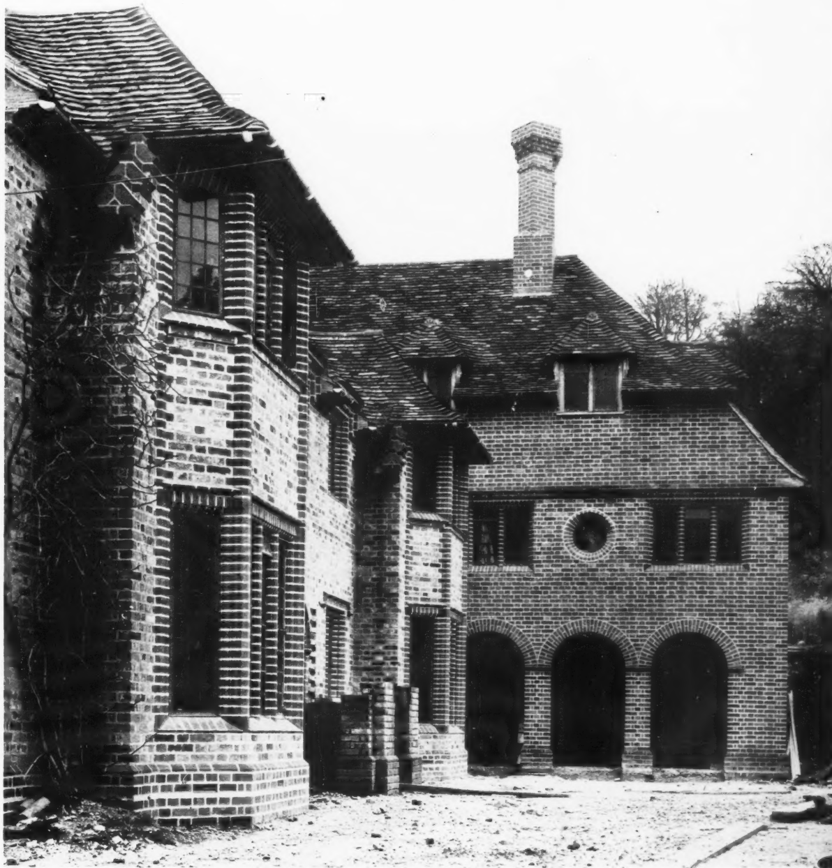
ENTRANCE FRONT IN COURSE OF REBUILDING
