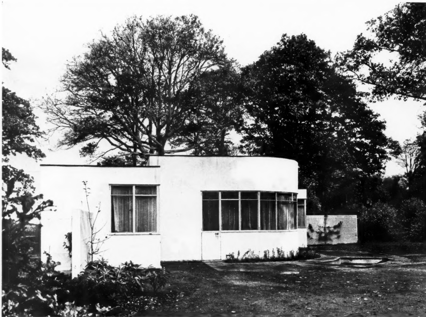
ONE-STOREY HOUSE on a site sheltered by trees on the north and open to fine views on the south. A tank room—often a problem in flat-roofed houses—is fitted in at a convenient break in roof level, where the height of living-room increases. The plan is a development of the basic "Sunspan" plan, exhibited at Olympia in April, 1934.
