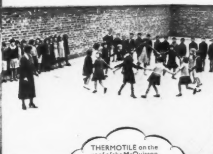
THERMOTILE on the roof of the McQuiston Public Elementary School, Donegal Place, Belfast. Used as a playground.
