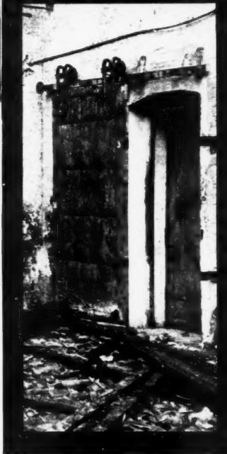
MATHER & PLATT HINGED & AUTOMATIC SLIDING DOORS AFTER WITHSTANDING A FIERCE FIRE
