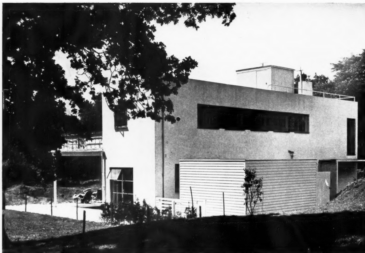
THE NORTH-EAST WALL, with the ground-floor nursery window on the left. The house is built for a composer, on the brow of a hill facing south in the hilly wooded country between Mere and Wincanton, on the borders of Somerset, Dorset, and Wiltshire. The music room, built among the trees at a distance from the house, is not illustrated here. The south front is constructed with a steel frame. Other walls are 11 in. hollow brickwork rendered and whitened. Window frames are painted light blue.
