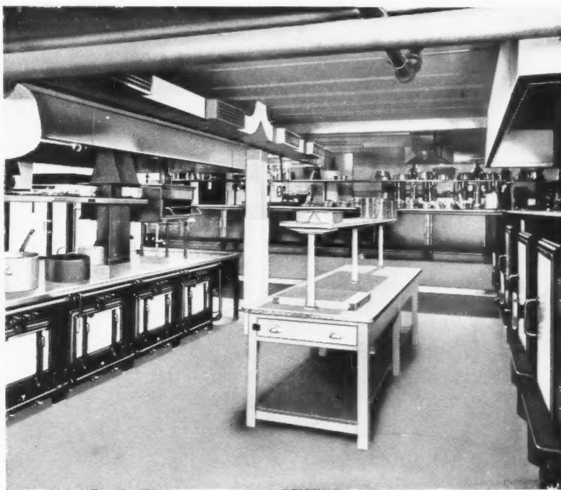
The gas-equipped kitchen at the London Casino
