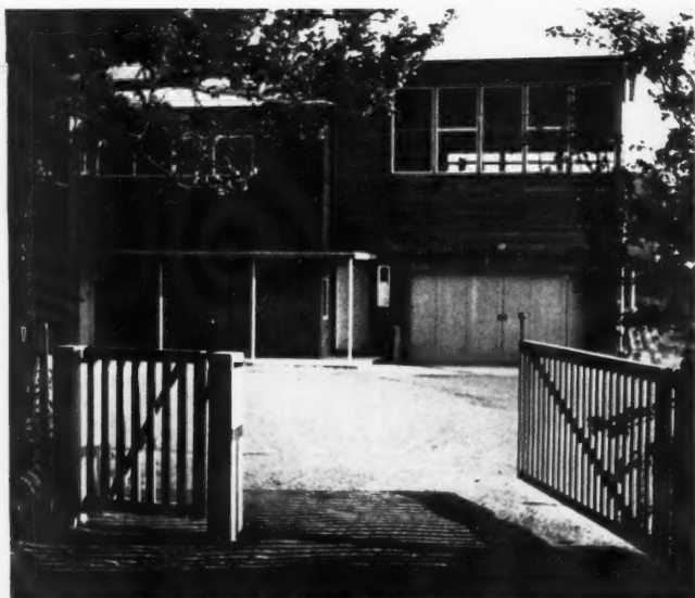
THE EXTERNAL STAIRCASE AND LANDING to the studio at first floor level, and below, the house as it is seen from the road, with entrance porch and the north window to the studio.
