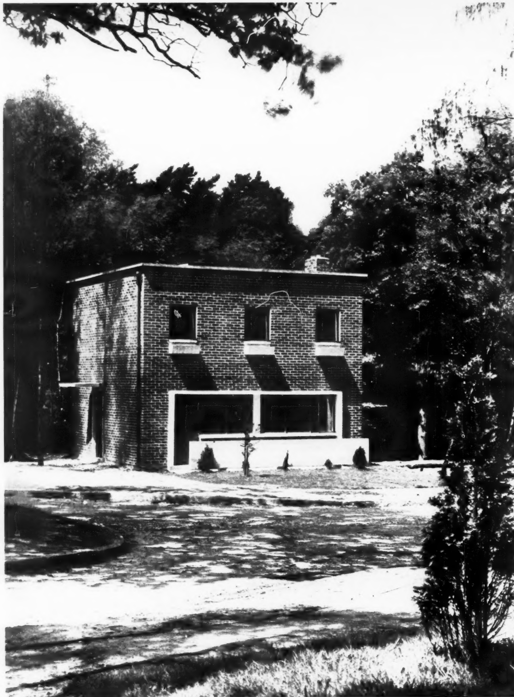
HOUSE TYPE B. Contrary to normal practice in speculatively built small houses which have the entrance at the front, with the hall at the side of a deep narrow living-room, the living-room here occupies the whole frontage, and the entrance is at the side. This accounts for an elevational expression of big balconies and windows with two bedrooms above, resulting in a resemblance to the eighteenth-century traditional façade.
