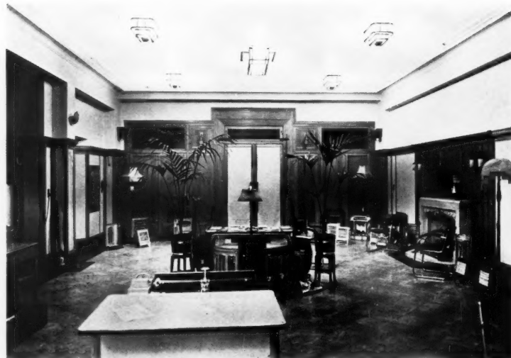
Dandee Corporation Electricity Showrooms. For the purpose of photographing, all lights in the room, with the exception of the G.V.D. units, were switched off. Notice the even distribution of light, and absence of glare, enabling the camera to record the details of the artistically designed ceiling boxes. Only one lamp is used in each.
