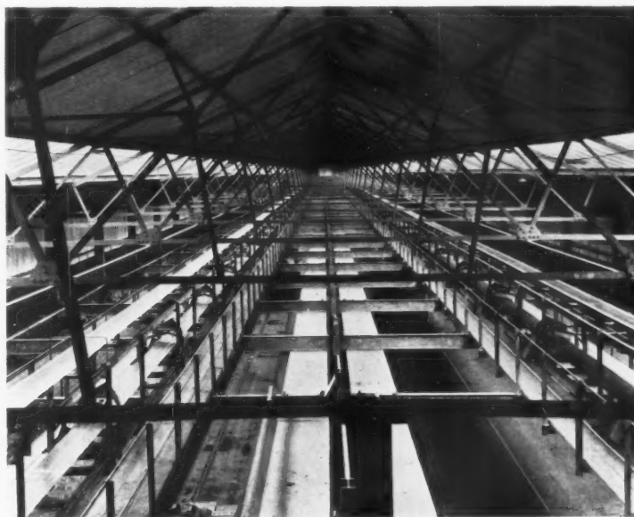
The five steel band conveyors at Ridgmont having a total length of 2,880 ft.—these conveyors feed the prepared clay into the brick Presses.
