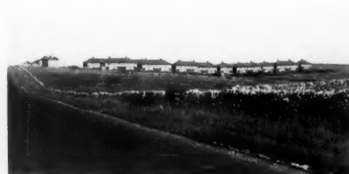
Fernilee: Industrial housing in the open country. Nature at their door makes these bad types of cottage endurable, but the opportunity for much more widespread building has been neglected.
