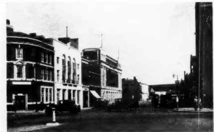
Uxbridge. New shopping streets as well as old display a riot of individuality in competing façades and a cacophony of advertisements: 10, Charles Street, Leicester: a new street driven through the centre of the town at immense cost.
