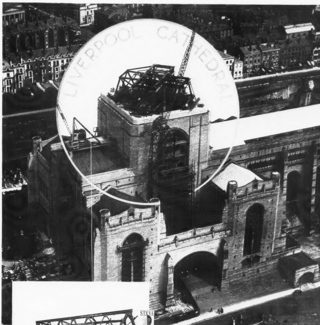
Aerial view of steelwork to support Bells and Ringing Chamber, etc., in the Tower, fixed approximately 200 ft. from ground level.
