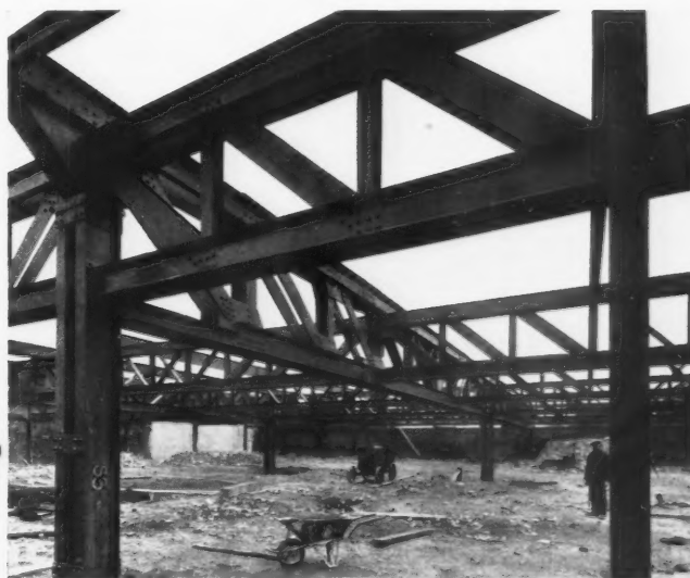
GARAGE—Steel Roof and Tennis Court Floor
