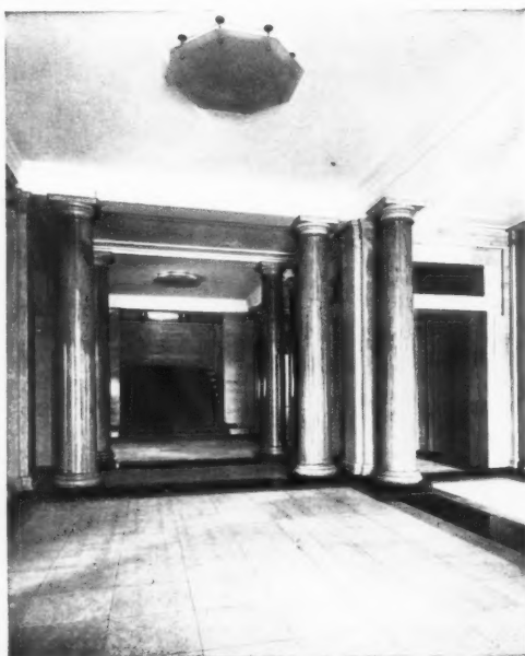
LEEDS CIVIC HALL.
