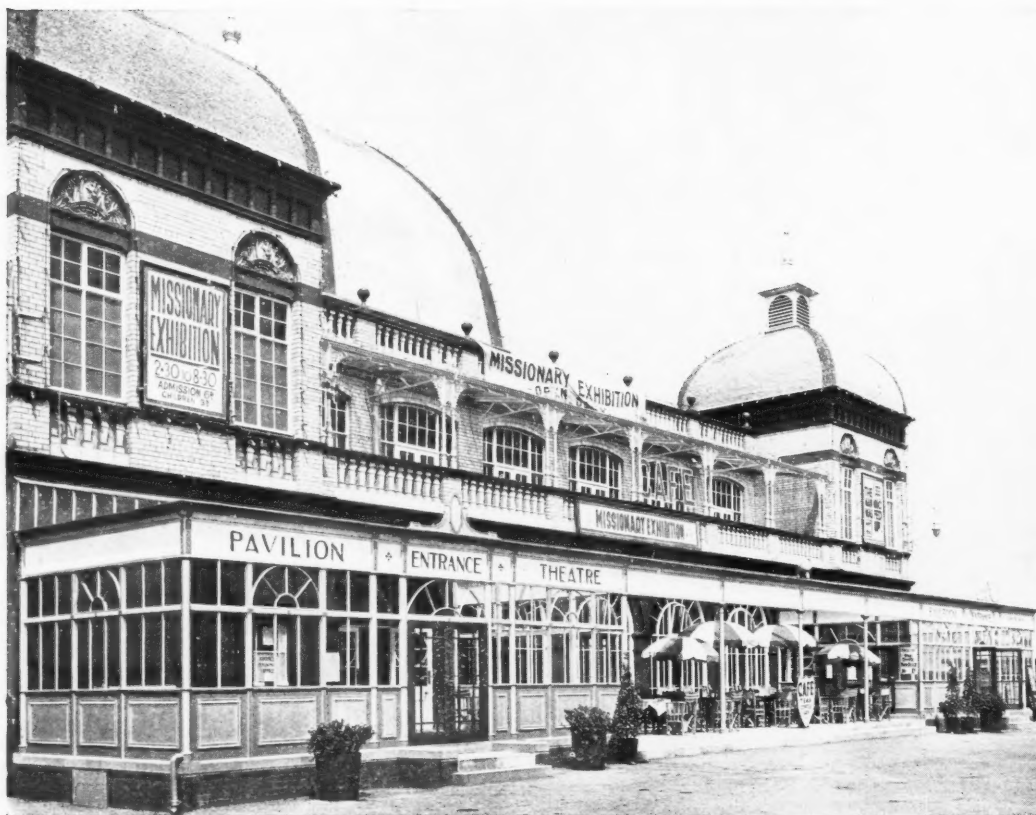
VERANDAH AND CRUSH ROOMS SUPPLIED AND ERECTED AT RHYL PAVILION. A. A. GOODALL, Esq., M.I.M.C.E., Engineer & Surveyor
