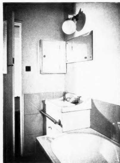
Bathroom equipment; lavatory basin with hot towel rail below, built into soiled linen cupboard. Designed by Frederick Gibberd.
