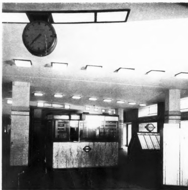
HOLBORN UNDERGROUND STATION BOOKING-HALL. L.P.T.B.
