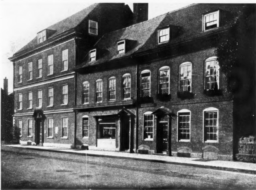
Throughout the seventeenth and eighteenth centuries the idea of the Street so informed the whole building tradition that even in the slow accumulative growths of the country towns, buildings generations apart in time stood together in a harmonious relationship of spirit. 5. The High Street of Yarm, Yorkshire. 6. Houses in Oxen Street, Hereford.
