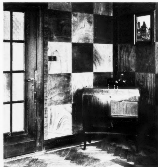
An example of Forssman wood panelling. The chequer-board effect is accentuated by crossing the grain of each alternate square.
