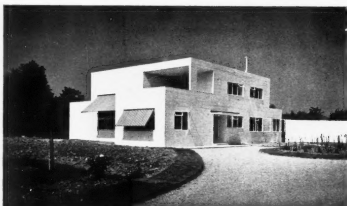
House at Nast Hyde, Hatfield. Architect: F. R. S. Yorke, Esq., A.R.I.B.A.
