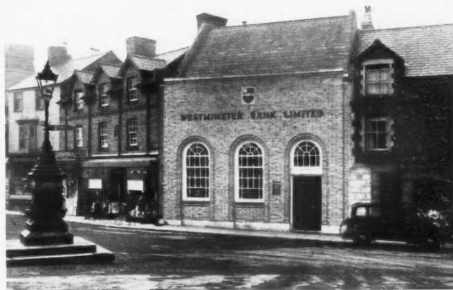
1. The Weston branch of the Westminster Bank. A. E. Shennan, architect.
