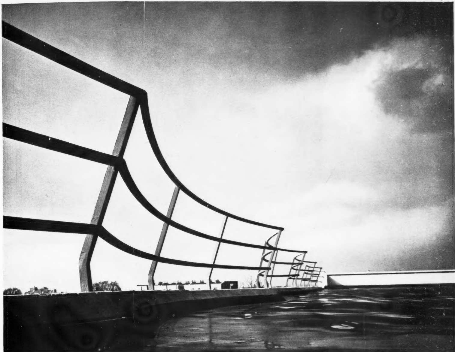
1. Fresh air and sunshine on the roof playground. The railings curve inwards so that it is almost impossible to climb up and fall over.
