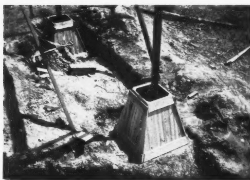
The concrete bases for the steel supporting columns in process of construction.
