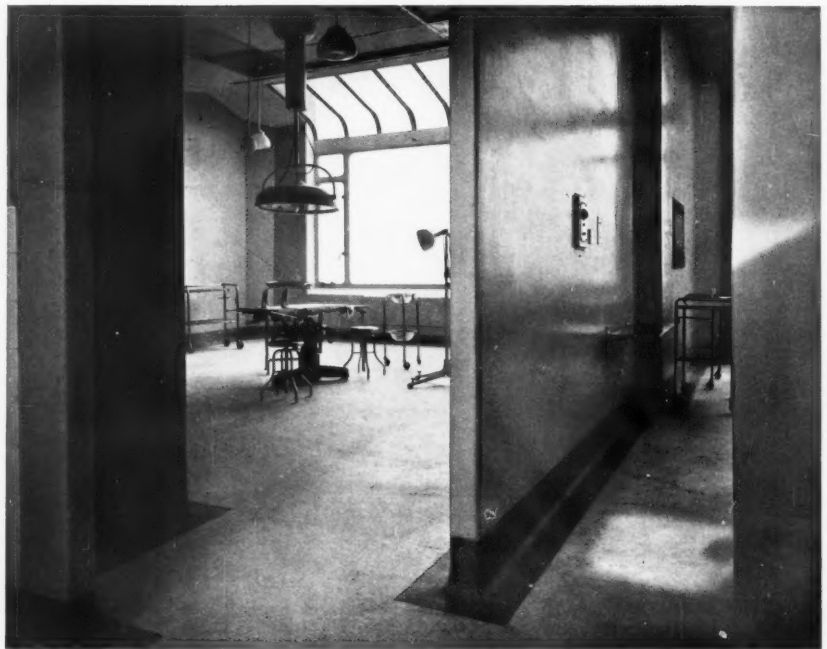
One of the operating theatres at the L.C.C. Hammersmith Hospital. G. Topham Forrest, architect to the L.C.C.
