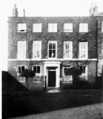
c.1825 "More glass than wall . . ." A house on Richmond Green. Maximum fenestration possible with supporting walls. Complete rationalization of form. "Architecture" has passed away. Amen.
