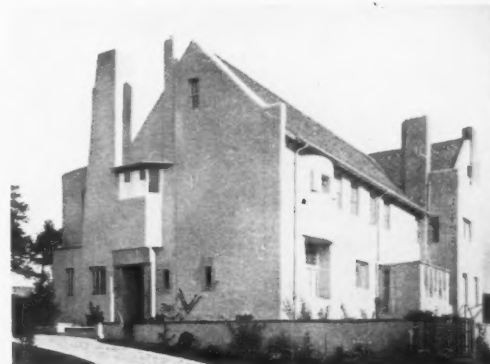
1911 C. R. Mackintosh's Hill House, Helensburgh. The false dawn of the new aesthetic, taking us back to the last example but one in all save non-essential. Clean surface and more light, but no structural advance; "art" is the prime motive.
