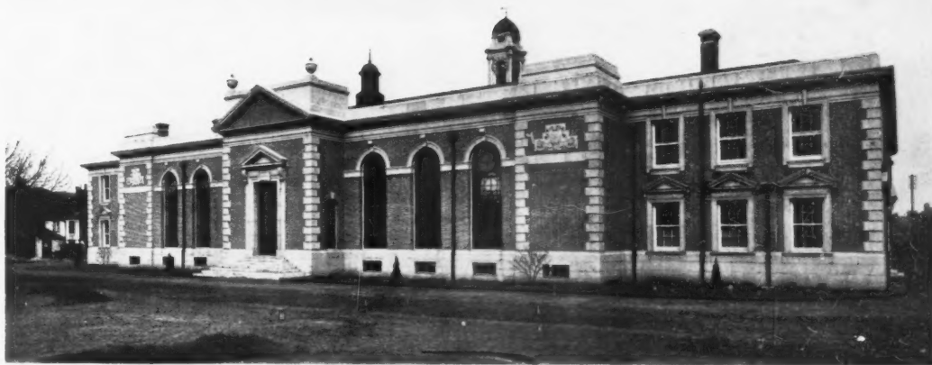
A. Grinberg, architect. 7. The Town Hall, Lewisham. Bradshaw Gass and Hope, architects. 8 and 9. The main and western fronts of the Town Hall at Bridlington, Yorkshire. P. Maurice Necton, architect.
