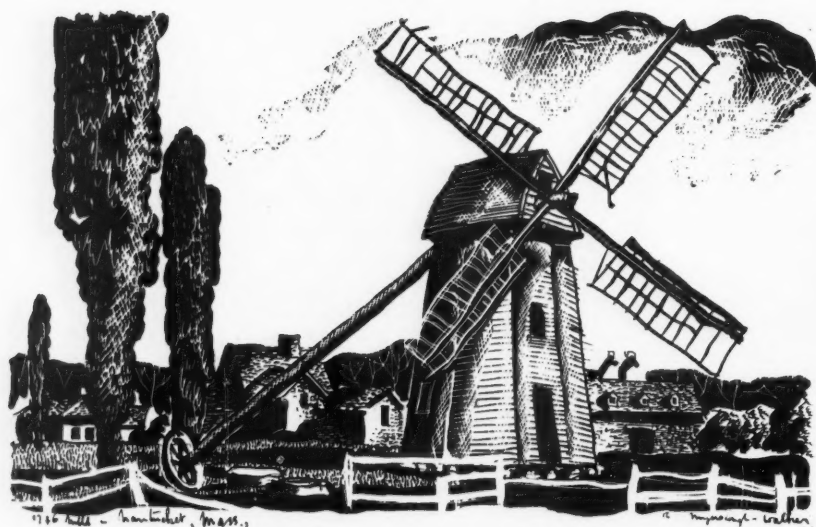
A smock mill at Nantucket, Mass., built in 1746 and differing from the smock mill common in Kent with its brick base and gallery from which the miller attends the sails.
