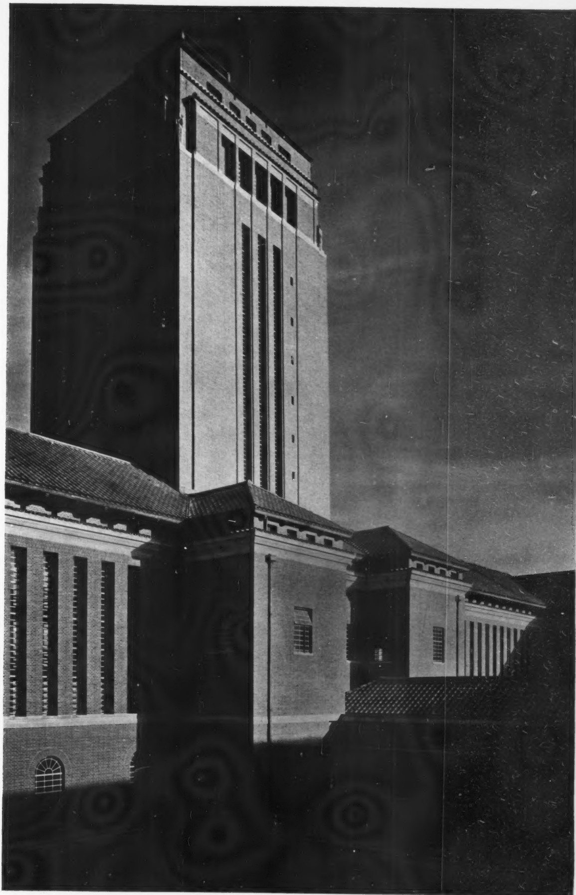
The tower of the University Library, Cambridge, from the north court. It is situated over the entrance hall and is fitted up as a vertical stack, which will probably be used for books that are not in great demand. The tower rises to a height of 160 ft.
