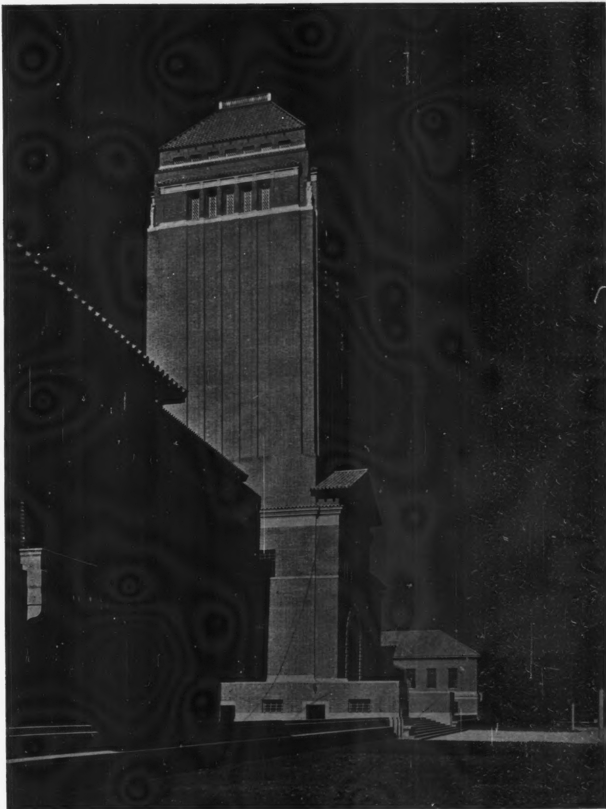
The principal (east) front of the University Library, Cambridge. The building stands on a comparatively level site, approached from Burrell's Walk, which branches off Queen's Road, and faces the western boundary of the new Clare College Memorial Buildings. The stone used on the exterior is a mixture of Clipsham and Weldon, and the colour harmonizes with the brickwork. The roofs of flat pitch are covered in Italian tiles of special design. Architect: Sir Giles Gilbert Scott.
