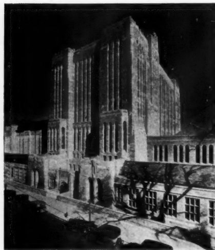
2. The new Stirling Library at Yale University. The books are stacked in the square tower, involving the loss of daylight. When further extensions are needed the height of the tower is increased. This American type of plan would, however, have serious drawbacks in open-access libraries like the University Library, Cambridge, where daylight is essential.
