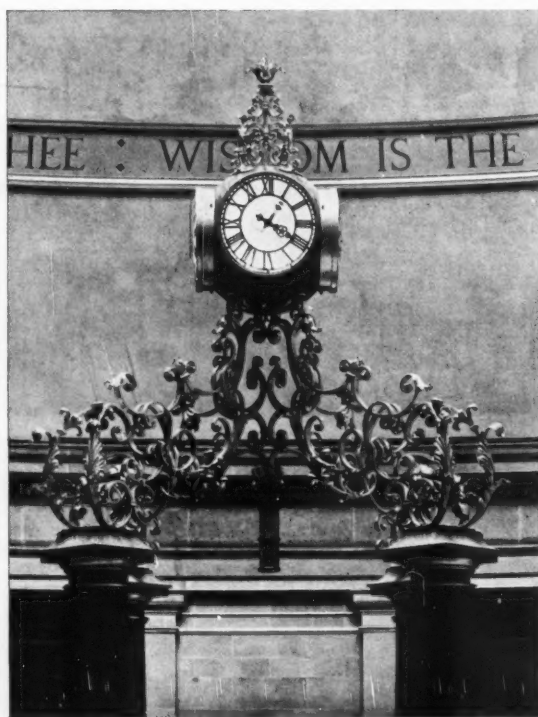
Clock case and wrought iron supports. Manchester Free Library. Architect: E. Vincent Harris, F.R.I.B.A.
