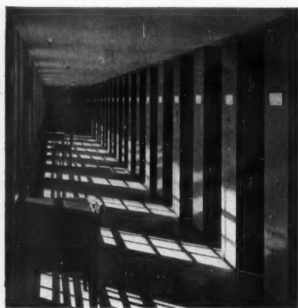
10. The bookstacks, the width of which is limited by the natural lighting from the windows.
