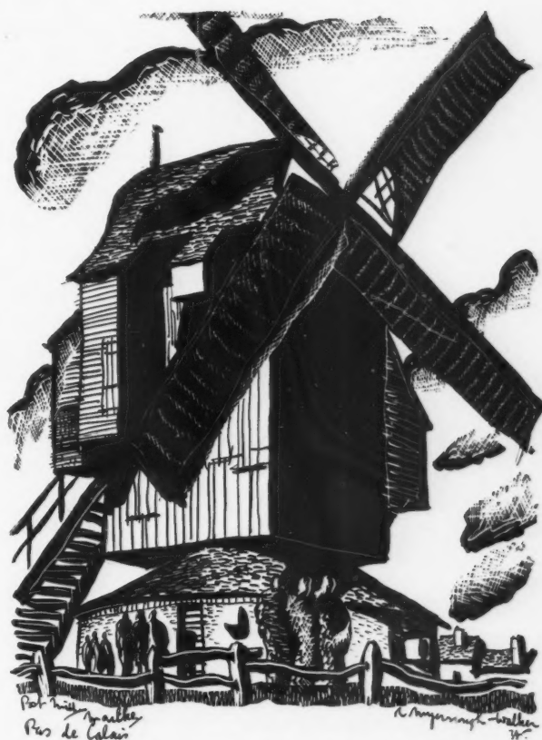
A post mill at Marche, Pas de Calais, fully sailed and a fine example of its kind. The projections house the flour dressing and other machinery and, incidentally, give to the structure a vigorous form almost monumental in its quality.
