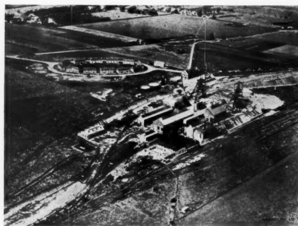
The beginnings of proper planning are shown in this aerial view of an East Kent works. The workers' dwellings are grouped separately, though they are not as far from the factory as one could wish.
