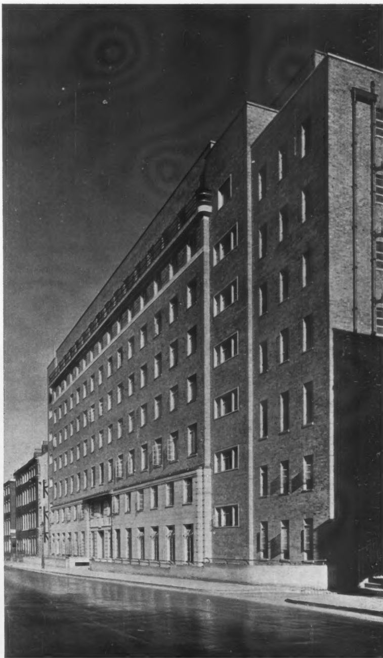
The principal elevation to Guilford Street and a detail of the Main Entrance. The sculptured panel was executed by Eric Aumonier.
