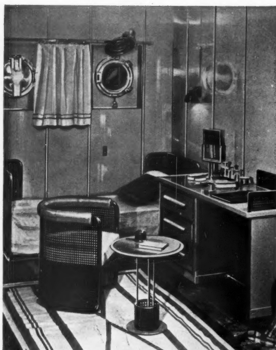
A complete ship's cabin, as exhibited at the Salon des Artistes Decorateurs, Paris. The walls are of aluminium alloy, with thermal insulation of "Alfol" (aluminium foil). The furniture and fittings are also of aluminium alloy.
