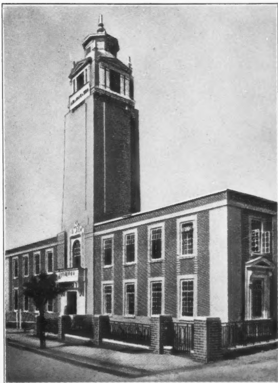
Photograph by courtesy of BUILDING.
