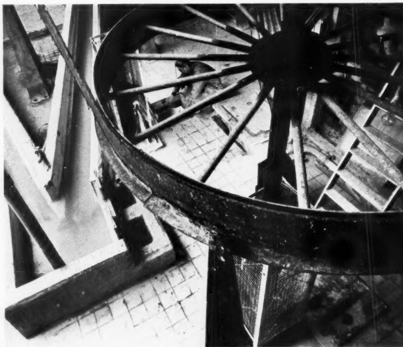
At Carter's Tile Works, Poole, Dorset: a view of the Slip House showing the foreman measuring materials into the mixing tank below floor level.
