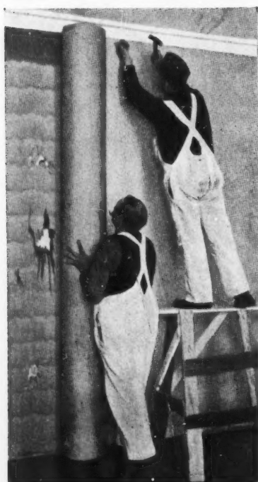
Tacking a roll of flexible wallboard along its top and bottom edges.
