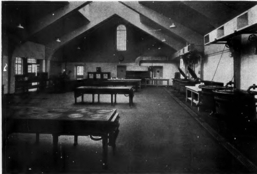
The kitchen of the Middlesex County Council Mental Hospital, Shenley. Appliances are electric and steam heated. Illustrated below is the all-electric cooking equipment of the Nurses' Home.
