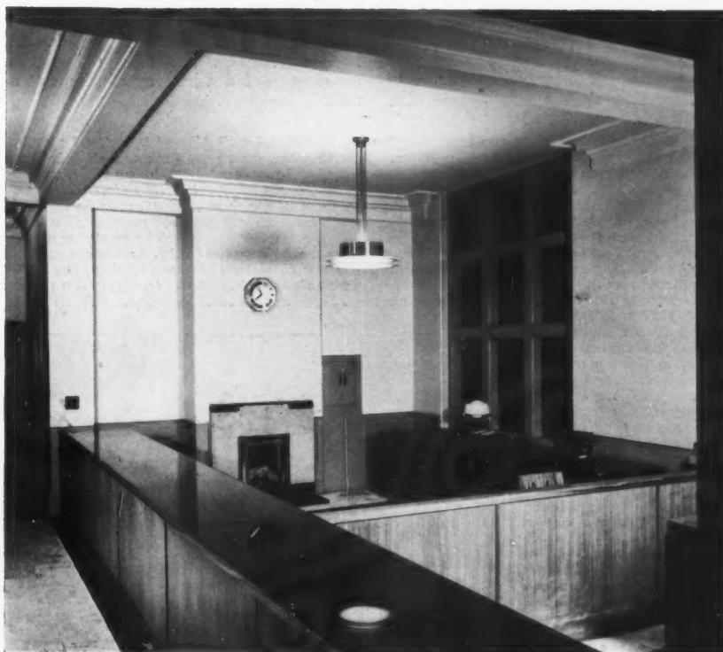
16. DEATH OF THE HOVEL: OFFICES WITH TRANSPARENT PARTITIONS. For a Steamship Company. The steel partitions are designed on the unit principle, a complete installation being carried out by the erection of a number of standard unit sections. Floor space in the modern office can be divided up with these partitions to give the greatest elasticity in design, and at any time they can be taken down and re-erected in some different lay-out, easily, quickly, and with an almost entire absence of damage to walls and ceiling. Architects: Meives and Davis.
