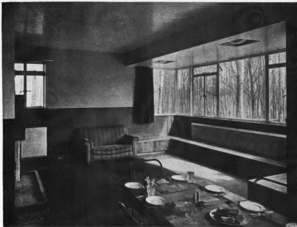
The "Lounge" end of the DINING ROOM of the new Boarding House, showing the window seats, with lockers under, in polished cedar. A dark grey linoleum floor and dado are surmounted with colours which vary according to the aspect of each wall. In this room lemon yellow and pale grey are used on the walls, the ceiling being white. The tubular steel chairs are finished in dark blue cellulose paint.
