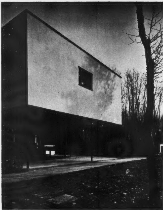
THE SOUTH END of the new Boarding House, showing the overhang which forms the "Covered Porch." This end has 11 in. cavity walls in a steel frame construction, supported on the 4 in. diameter steel columns in the foreground.
