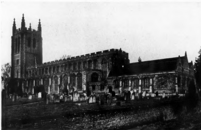
HOLY TRINITY CHURCH, LONG MELFORD, showing the eighteen clerestory windows on the north side urgently in need of restoration.
