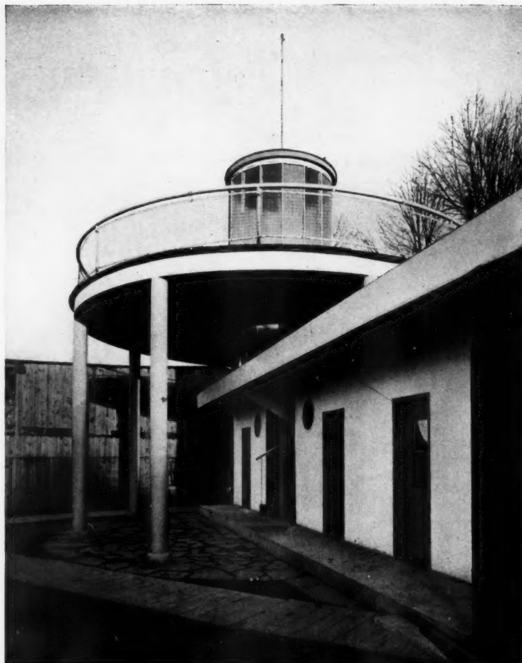
5. Another view of the terrace showing how the sloping roof serves as a protection to the lower part of the building.
