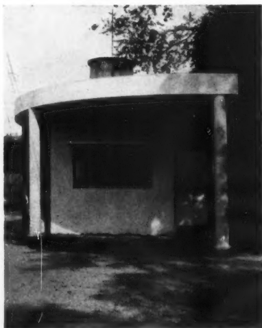
6. The refreshment room has movable glass doors on two sides leading out under the roof. Refreshments are served
