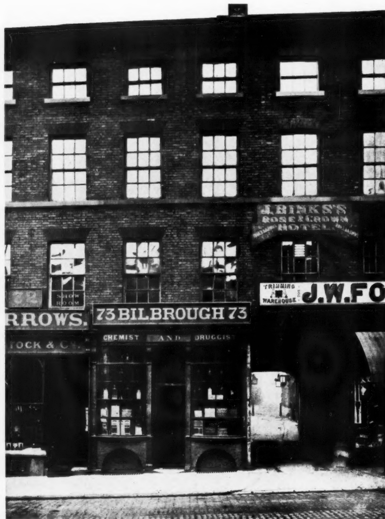
The old Commercial tradition of Leeds, illustrated here, makes an interesting comparison with modern commercial Leeds illustrated on pages 136 and 137 of this issue. This photograph was taken many years ago where Queen's Arcade now stands.
