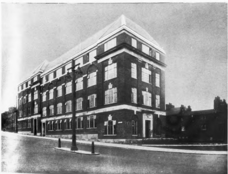
THE HEADROW, at its eastern extremity. The beginning of the block to be continued up the hill. In the foreground is the Kingston Unity Friendly Society (architects: Kirk and Tomlinson). The further part of the building is Messrs. Wharram's Warehouse. Architect: G. W. Atkinson.
