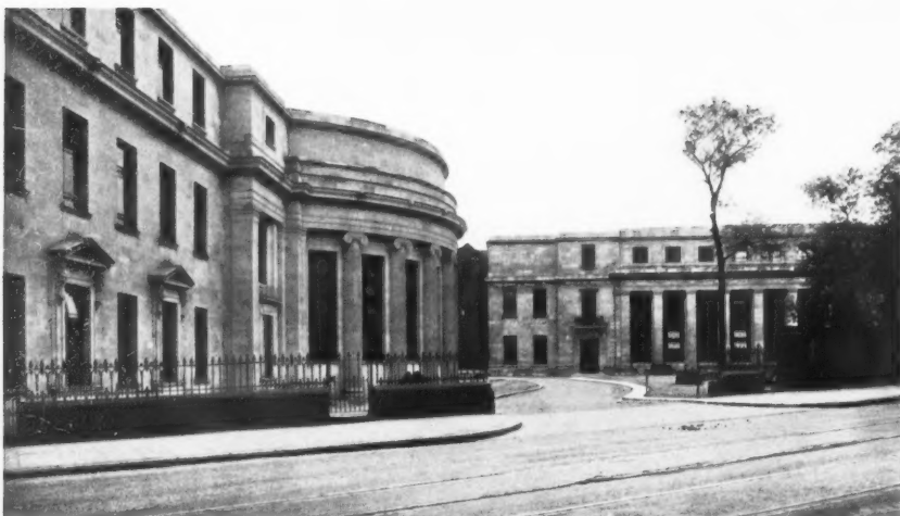
A general view of the hitherto completed work taken from Woodhouse Lane showing the chemistry block
