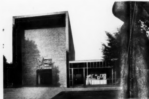
Detail of the entrance front and a back Architect : Ballo.
