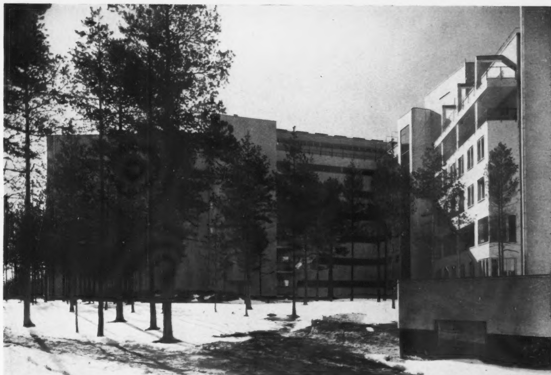
1. North view, under snow, of the balconies and (in the right hand corner) the nurses' rest-rooms (WING B, 4 on the second floor plan). In this wing all the nurses sleep, except the matrons. The back wall of the "lying hall" for the more serious cases can be seen on the left-hand side.
