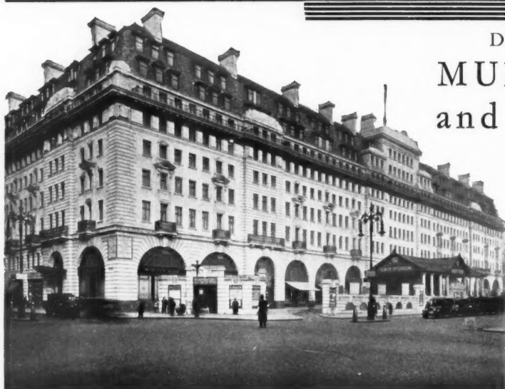
In this imposing building, Chiltern Court, Baker Street, London, W., Dockers' MUROLEUM Flat and SYNTHOLUX Gloss Paints for re-decoration have been used. The Architect is Charles W. Clark, Esq., F.R.I.B.A. (Metropolitan Railway, Baker Street Station), and the Painting Contractors, Messrs. John Laing & Sons Ltd., Mill Hill, London, N.W.7
