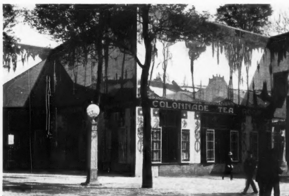
Outdoor 'atmospherics' in glazed concrete. A RESTAURANT.
