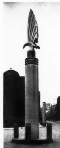
The pylon, which stood at an important cross roads at Liverpool during the Railway Centenary celebrations. Architects, W. G. Holford and G. Stephenson. A model of this in stainless steel has been presented to Professor Reilly.
