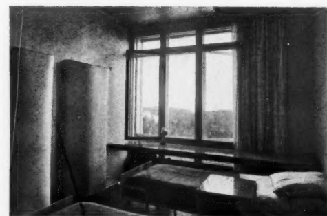
17. A standard two-patient "ward." The fresh air ventilation is between the double windows.
