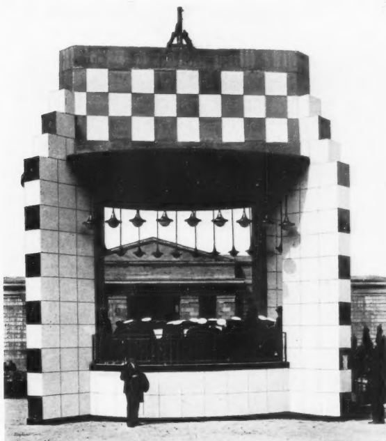
A BANDSTAND of cement blocks glazed and painted.
