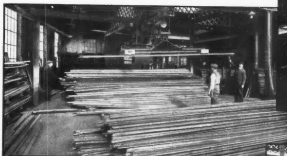
A Corner of the Bar Material Stores
