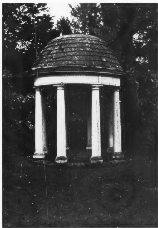
garden the original cupola serves as a summerhouse. The owners of the latter can hardly be blamed for not wanting the former.
