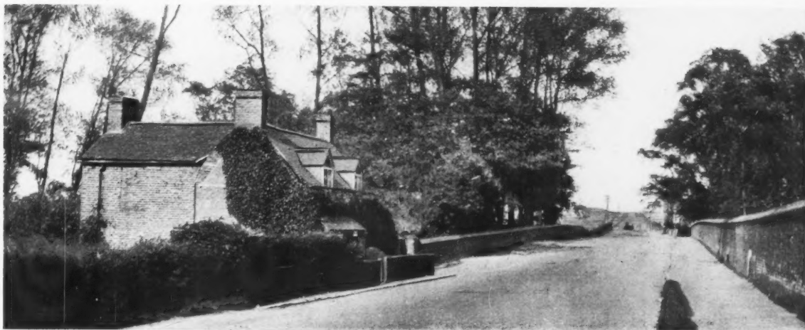
AS IT WAS: Wollaton Road, Nottingham, as it appeared ten years ago.
