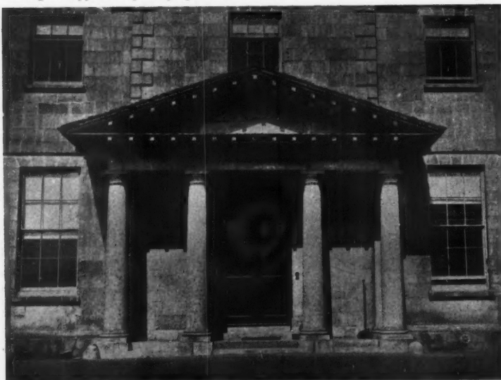
4. The entrance porch on the south front, Glynn. This, with its four monolithic Tuscan columns of granite, was probably added in 1820. The house was built in 1805 and was burnt out inside in 1819.
