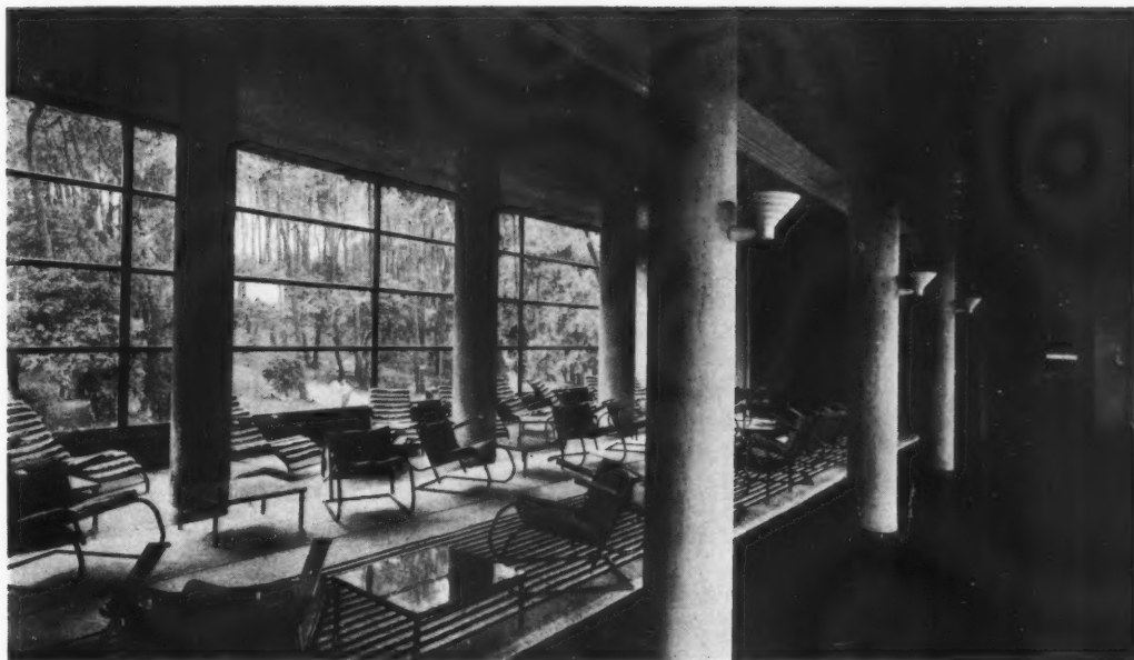
12. The hall (see No. 8, first floor plan) with its two long walls entirely of glass.
