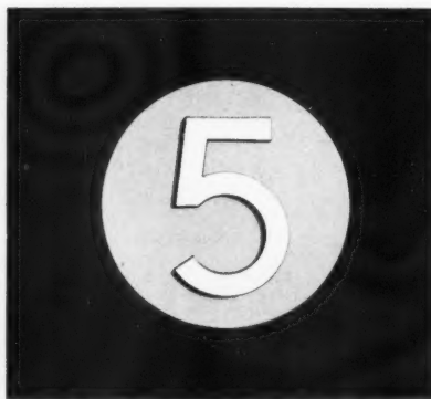
A floor indicator at Broadcasting House. Cream on a black laminated Erinoid figure on a red wooden block and a shallow black box which opens on a side hinge to reveal a complete list of offices and occupants on that particular floor.
