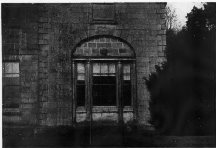
5. The library window on the eastern projection of the south front, Glynn. This detail shows the influence of Wyatt who was at work in Cornwall in 1805 and built St. Kea Church in the county in 1802.
