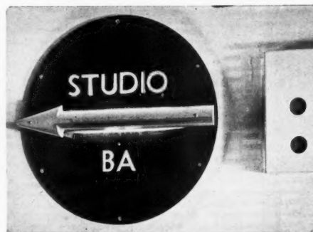
A wall directional sign in the waiting room of the vaudeville and dance band studios of Broadcasting House. The illuminated arrow is lit from behind. On the right is a portion of the artists' call indicator, which flashes the cue number to the performers awaiting their call.
