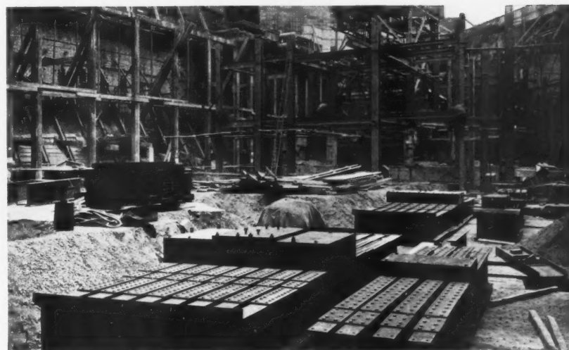
90 A large steel "bloom" in position on the grillage. This piece of solid steel weighs approximately seven tons and will distribute a load of over one thousand tons from one of the stanchions carrying large plate girders in Studio No. 1 that will be superimposed upon it. In the foreground to the right can be seen the rivet heads of the lower grillage that has already been grouted with concrete.
