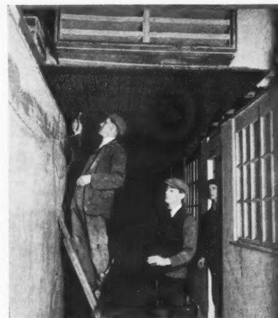
91 Corridor ceiling construction. The method of sound-deadening ventilation trunks is clearly shown.
