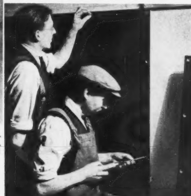
63 Fixing synthetic resin sheets, veneered on plywood, in studio B.A.
