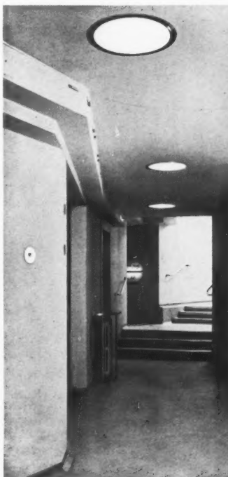
72. The 8th floor corridor leading from the lifts to Studios 8A and 8B. This corridor was lowered to accommodate pipes and conduits. Comfortable head room was maintained by a system of sunk lights flush with the ceiling. Walls are pale yellow, floor cream coloured composition.
