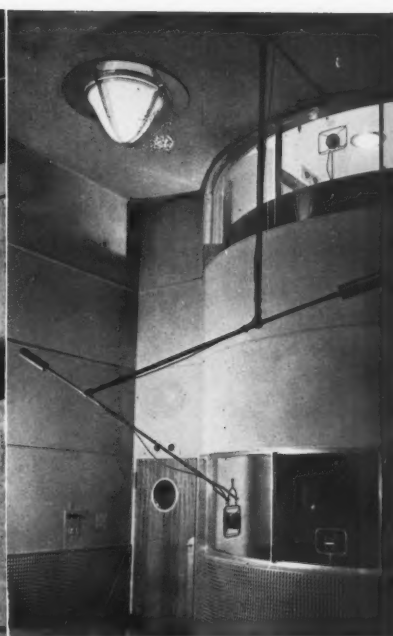
110 Dramatic effects studio, showing the ingenious doubly counterbalanced arm microphone fitting. The cable is attached to the arms by open clips, and the weight of different microphones is balanced by a fine screw adjustment on the weighted ends of the arms. The microphone can be moved to any desired point in the space of the room and remain there perfectly balanced, thus freeing the floor space of stands and cables.
