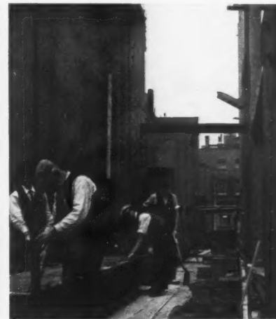
92. On the left are the ten-foot six plate girders and mass brick wall of the studio tower—the isolating corridor—with the steel frame of the office block on the right, structurally separate from the studio tower.
