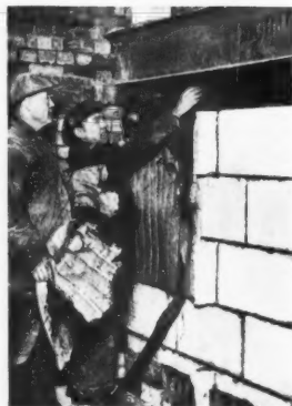
94 The partition walls of cellular concrete blocks with eel-grass sheets sandwiched between.
