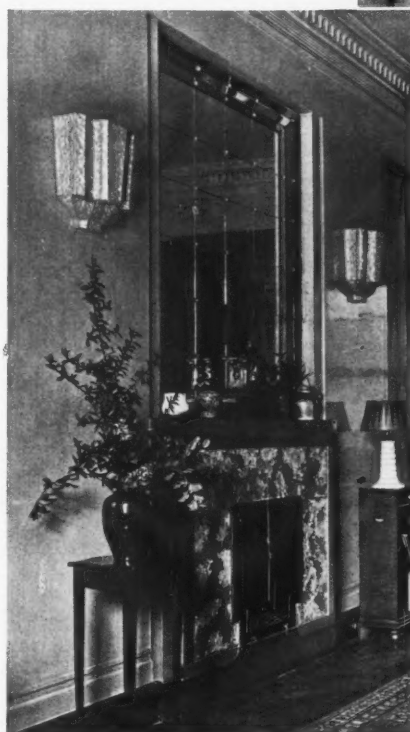
A GAS FIRE WITHOUT A HEARTH. The asbestos heating tubes are concealed by a pair of folding lids when the gas fire is not in use. The illustration is of the drawing-room of the late Sir Lawrence Weaver who did much to improve the design of gas fires.
