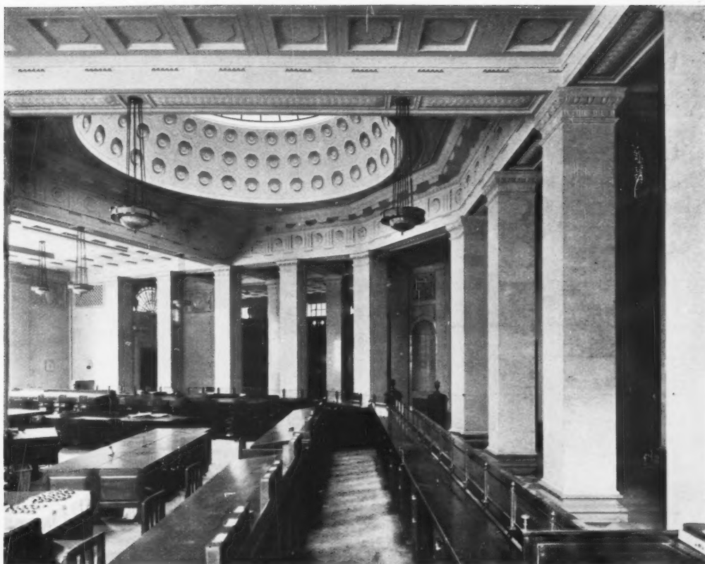
THE BANKING HALL.—The walls and columns are built of Subiaco marble. The floor is in Roman stone and the ceiling in fibrous plaster. The counter is made of teak with a Sienna marble and bronze front. The desks are in teak.
