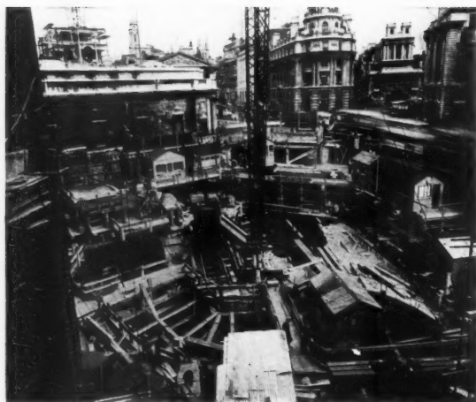
THE FOUNDATIONS IN PROGRESS. Three sectional iron caissons 40 feet in diameter were sunk in the centre of the site to a depth of about 55 feet, and in these, large stanchion bases were constructed and the stanchions placed in position. Small borings were then made between the caissons and the outer walls, and the cross steelwork was threaded through and the whole of the steel frame structure completed.
