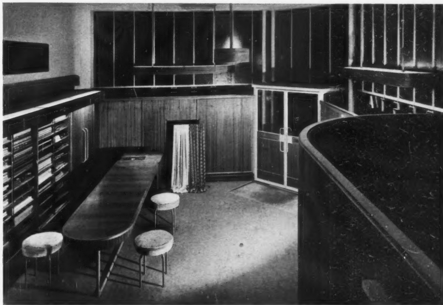
SAPELE MAHOGANY VENEERED PLYWOOD, AND LAMINATED BOARD, with a solid mahogany recessed capping, form the curved partition seen in the lower right-hand side of this photograph of a Cresta silks shop at Bromley, Kent.
