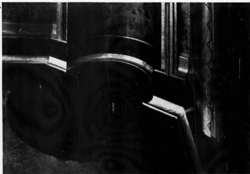
Dark polished BURR WALNUT on PLYWOOD covers the walls of this room at Bechstein Hall, Brook Street, London, designed by Sir John Burnet and Partners. The skirting is Zirracotti veneer with a dark, almost black, streak. The cove of walnut gives a definite break between wall and floor.
