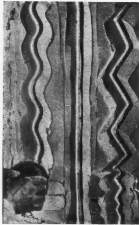
The ease with which PLASTIC PAINT can be manipulated, and how, by a slight movement of the hand, three different patterns are formed from the same tool, is shown in this illustration.
