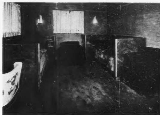
LAMINATED BOARD with a sycamore veneered face lining the "walls" of a first-class cabine-de-luxe on the s.s. Campana .
